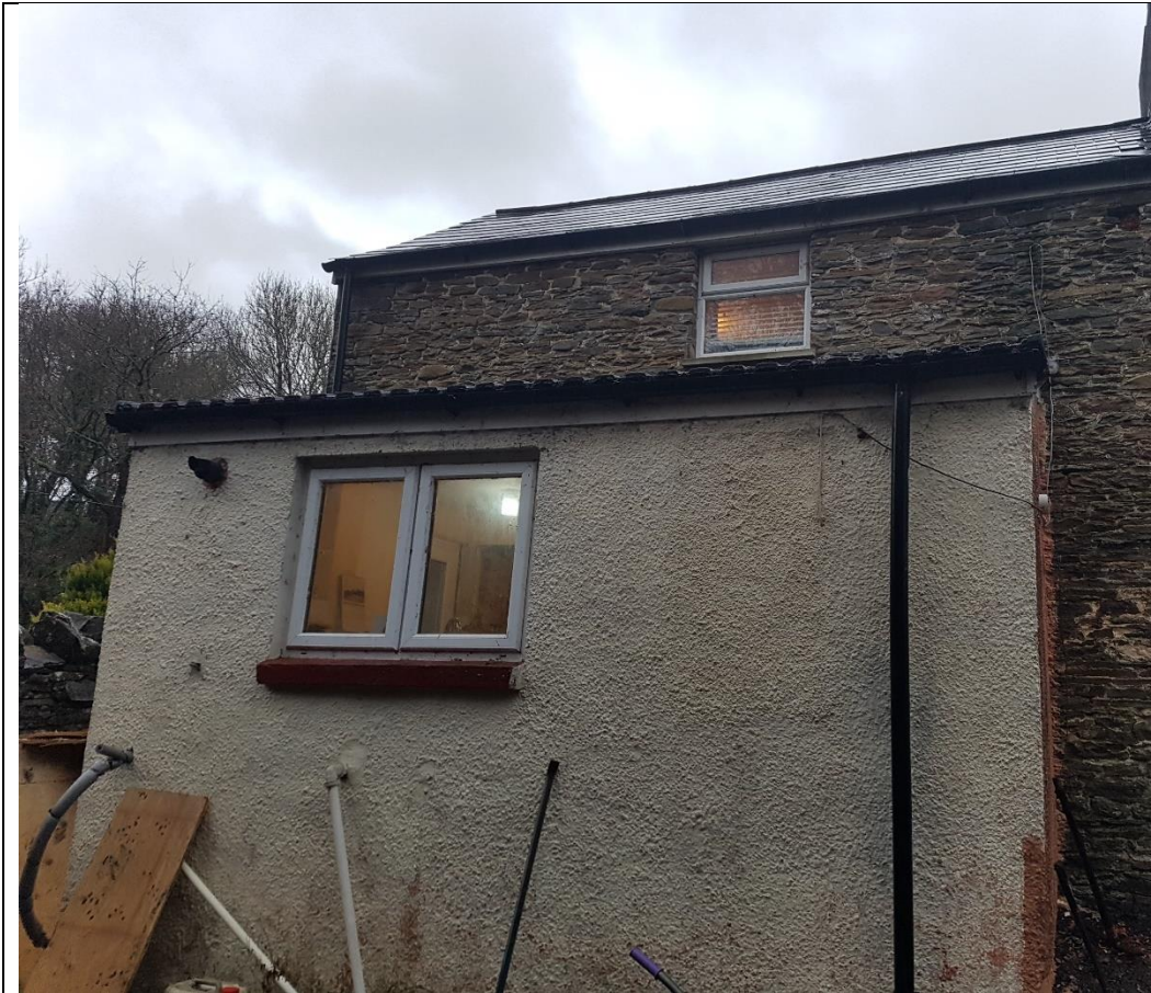
Photo 2. Rear (west) with lean -to for demoliti on
