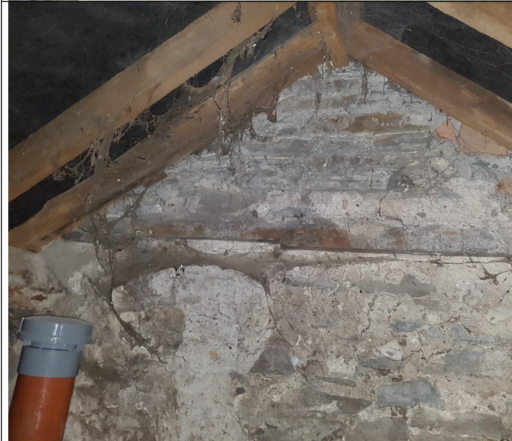
Photo 9. Interior of cottage loft including gable end
