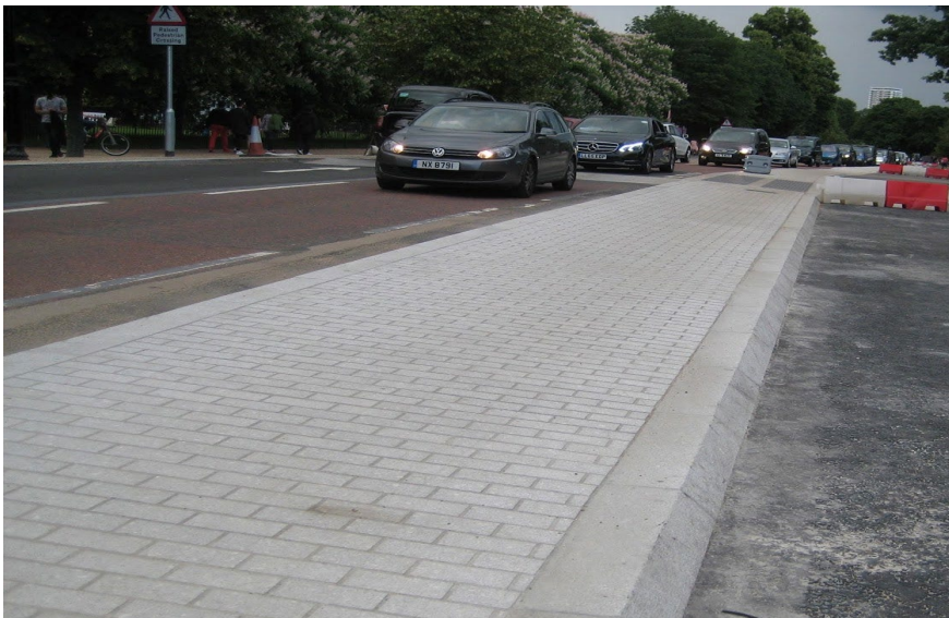
Paved crossing points in car park
