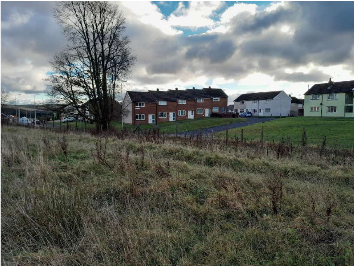
Image EDP A1.7: South-east facing view of the central southern edge of the Site. Image to show the location for the 1901-1905 depicted boat house on historic OS Maps ( Plan EDP 5 ). Heritage walkover identified no extant remains associated with the former boat house.
