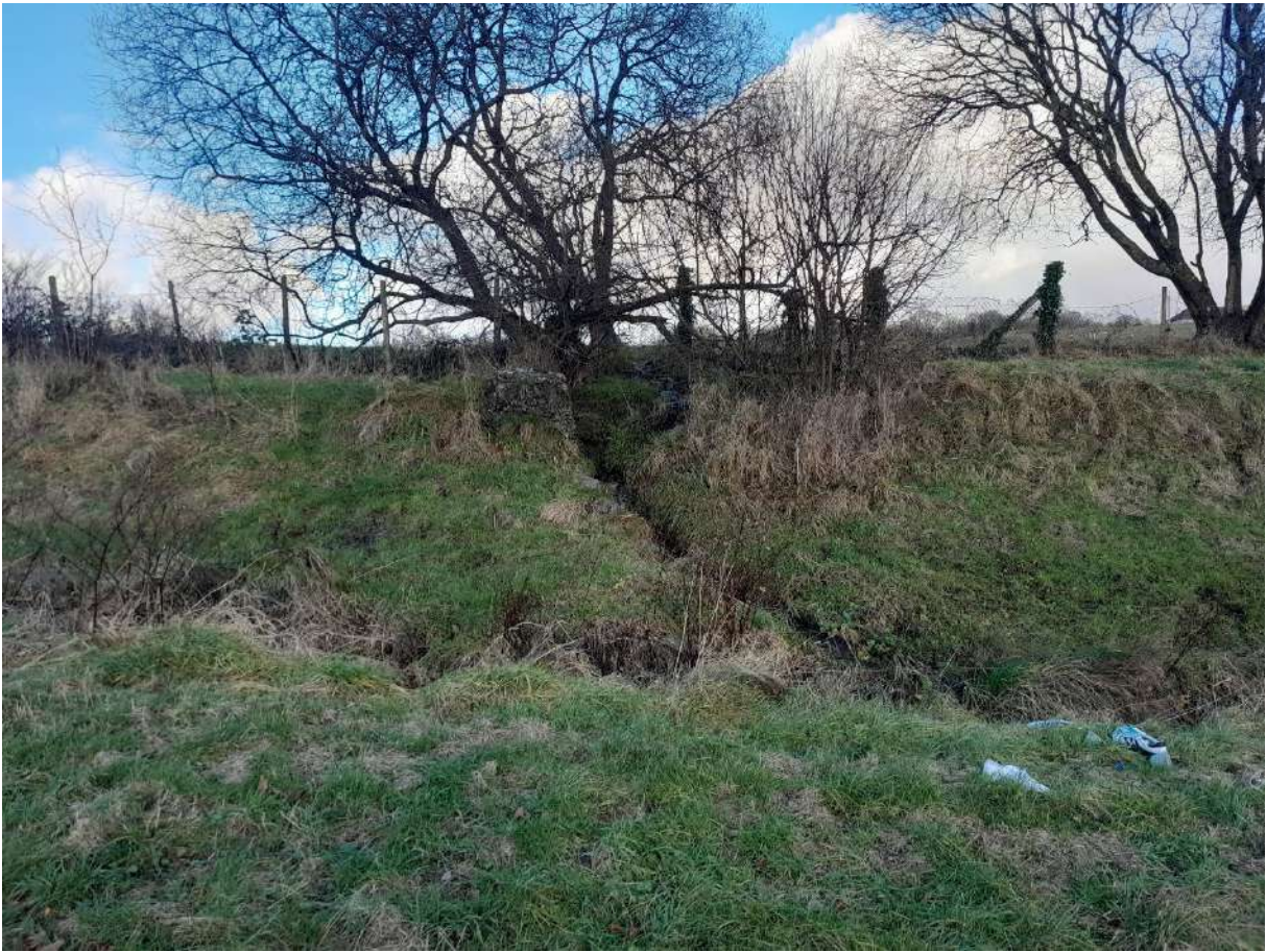
Image EDP A1.6: North facing view of the sluice gate remains to the former 'Goitre Pond', located beyond the south-east Site boundary. Remains of the west side stone abutment are visible.
