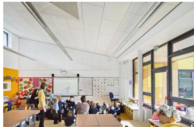
Figure 2: Acoustically absorptive mineral fibre ceilings
