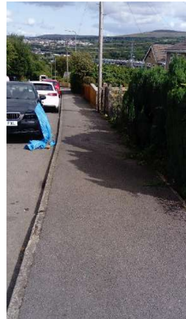
Plate 3.4: Footway along eastern side of Graig Road
