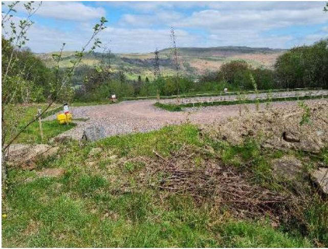
Figure 15 – View south across new car park area.
