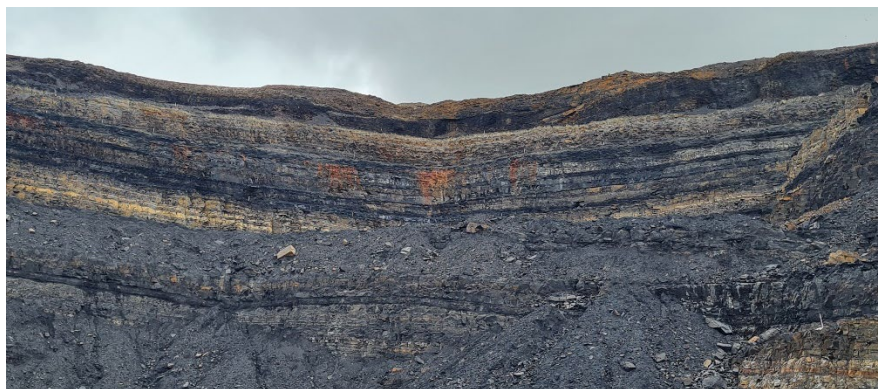
Figure 2 (top and bottom) Staining (orange) seen at seepages from 'R' seam
