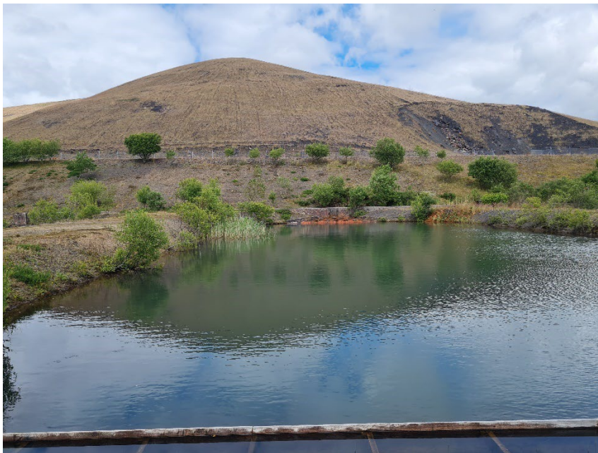
Figure 12 Sediment ponds showing orange staining at northern end.
