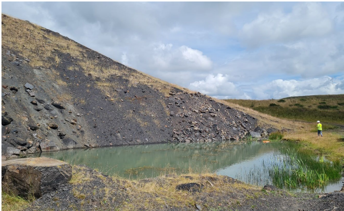
Figure 8 Pond at the toe of OB3.
