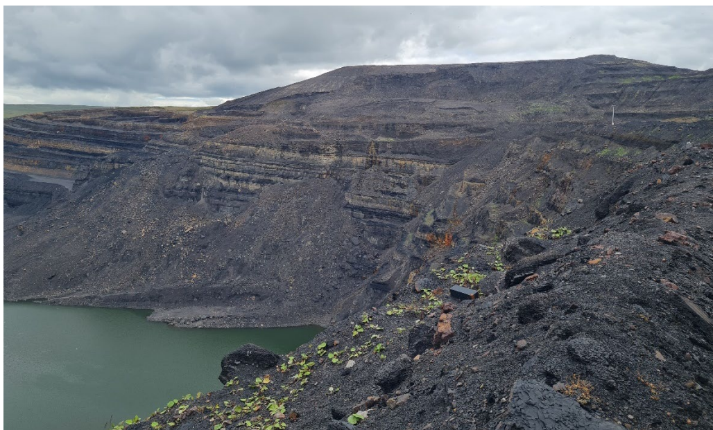
Figure 3 Eastern wall fail and OB1 slumping
