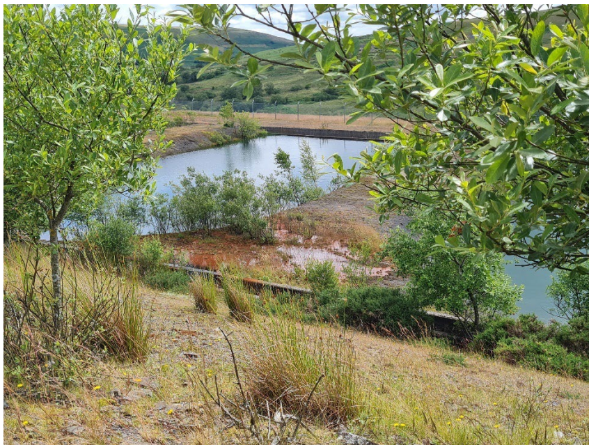
Figure 13 Concentration of orange staining around leaking Penstock valve.
