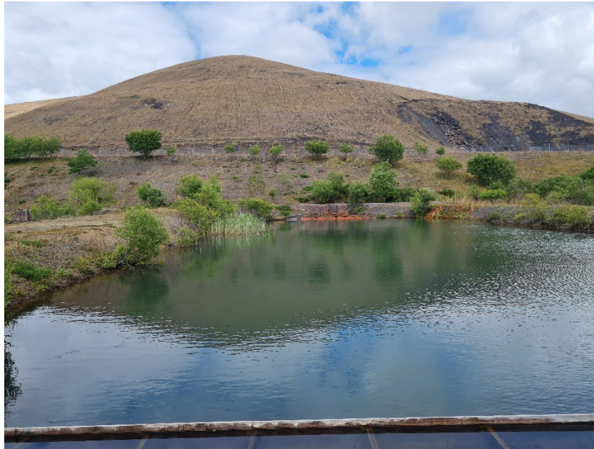
Figure 9 Sediment ponds showing orange staining at northern end.
