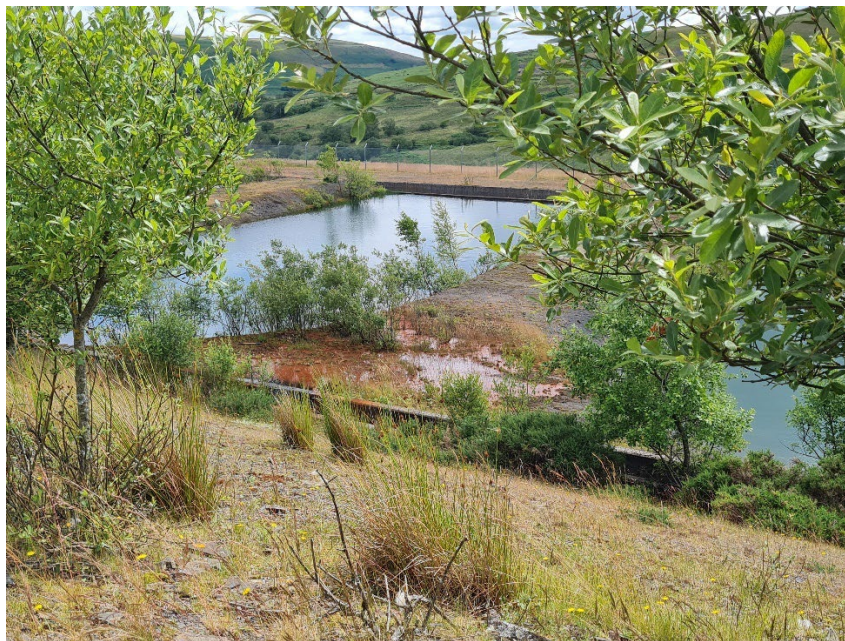
Figure 10 Concentration of orange staining around leaking Penstock valve.
