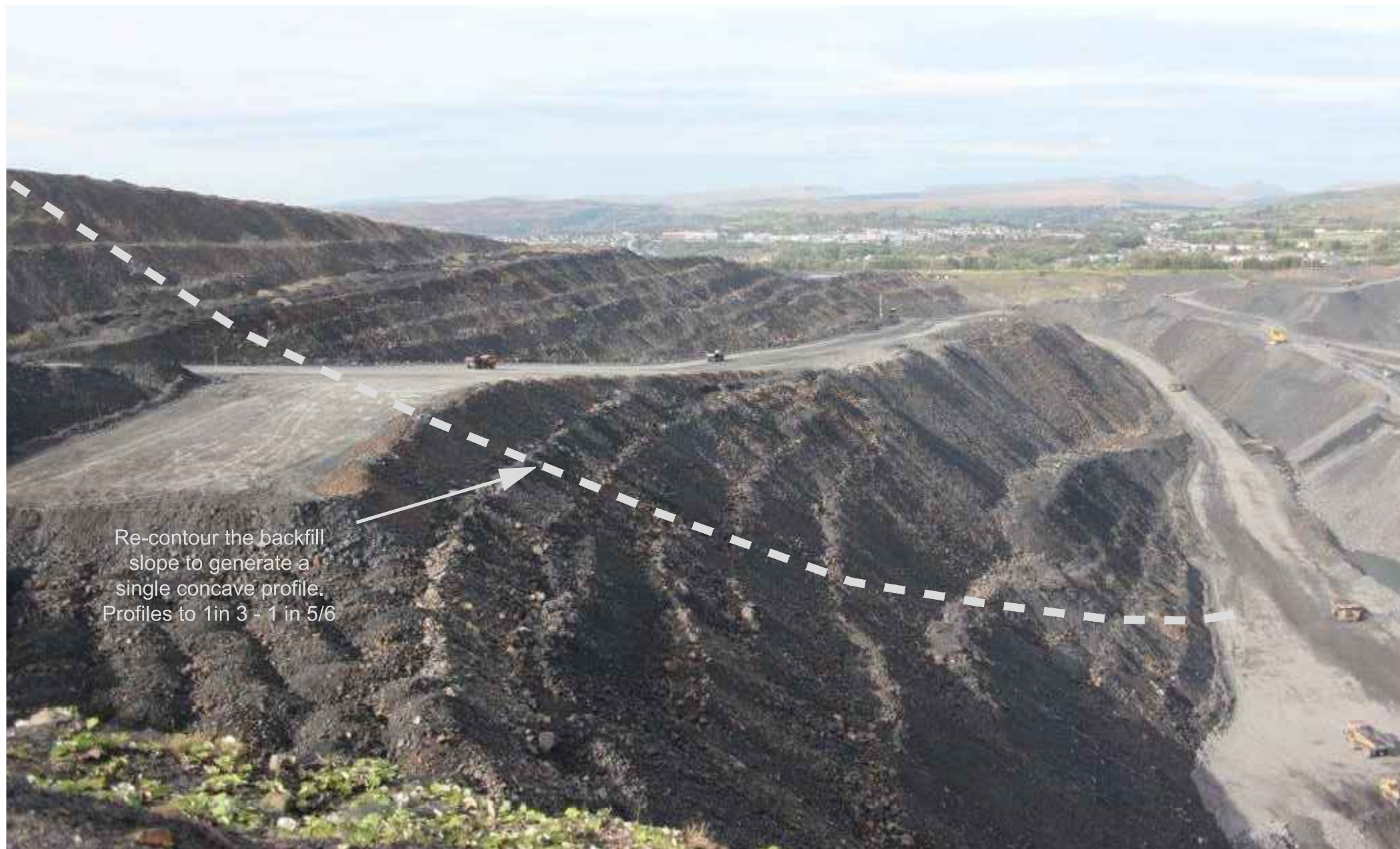
Drawing No 4 - Backfill ( Looking North)
