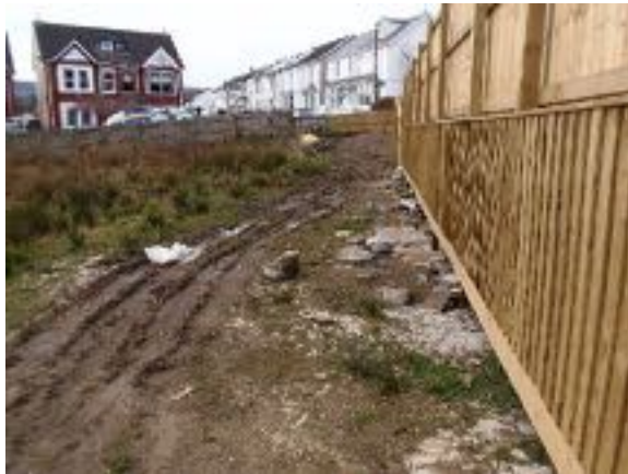
Site looking west along north west boundary
