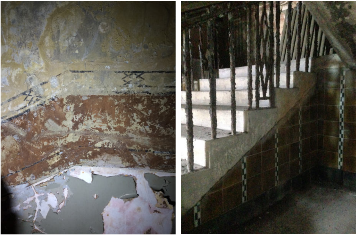
A 565.9 EXISTING CONDITION SITE PHOTOGRAPHS
