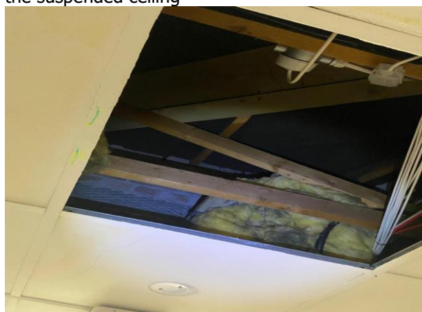
Photo 14: View into a section of the loft void above the suspended ceiling
