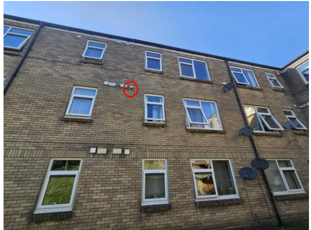
Photo 6: Missing mortar on western gable
