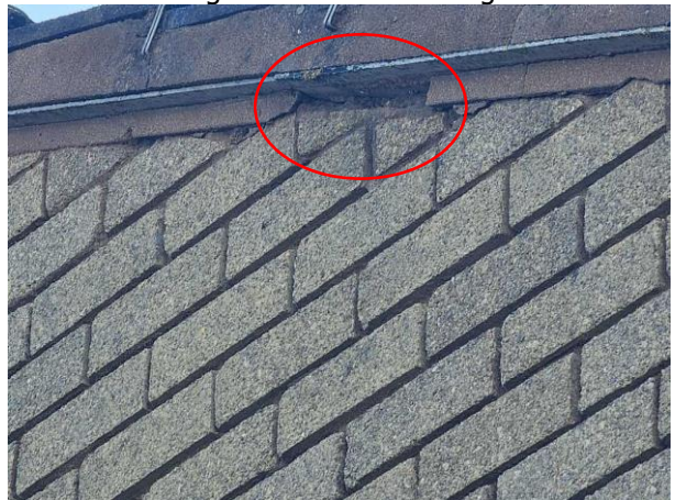
Photo 6: Missing mortar on western gable
