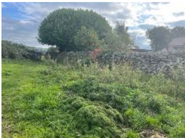
Photo 1. South boundary of site. Dry stone wall.
