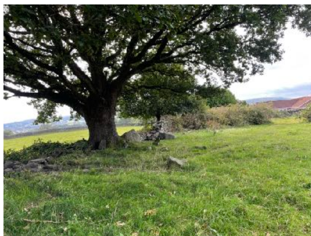
Photo 6. East boundary of site. Dry stone wall fallen in places with scattered trees.
