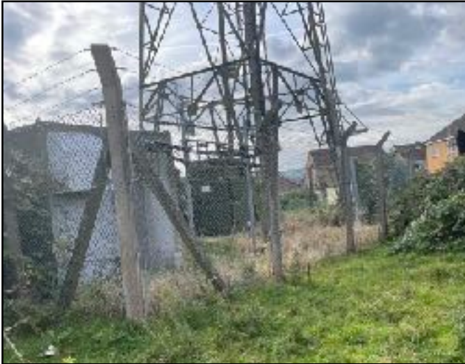
View of buildings and mast
