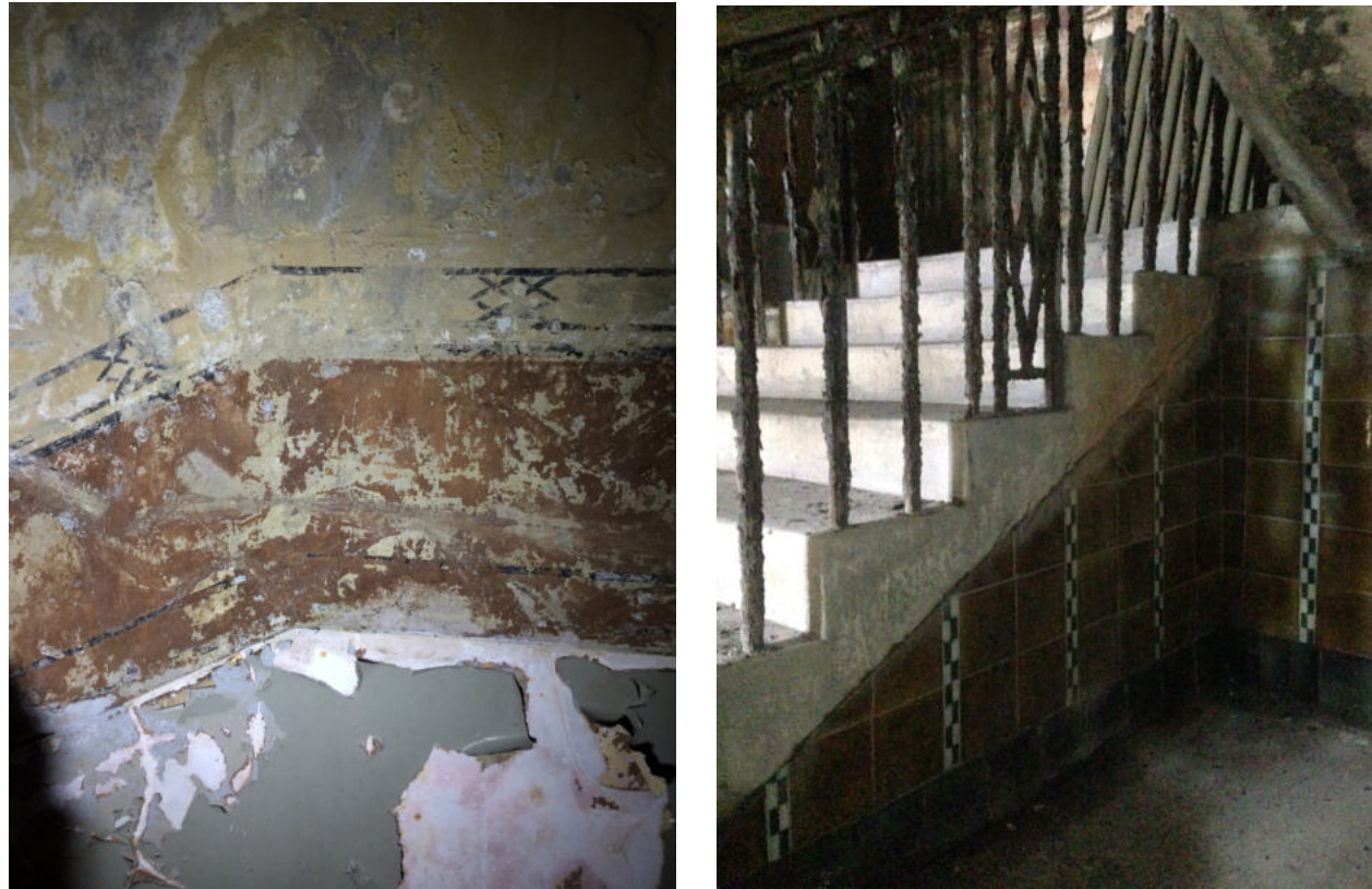
A 550.3 EXISTING SITE PHOTOGRAPHS
