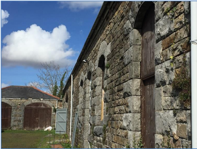
Photograph 25. Building F. The southern elevation.
