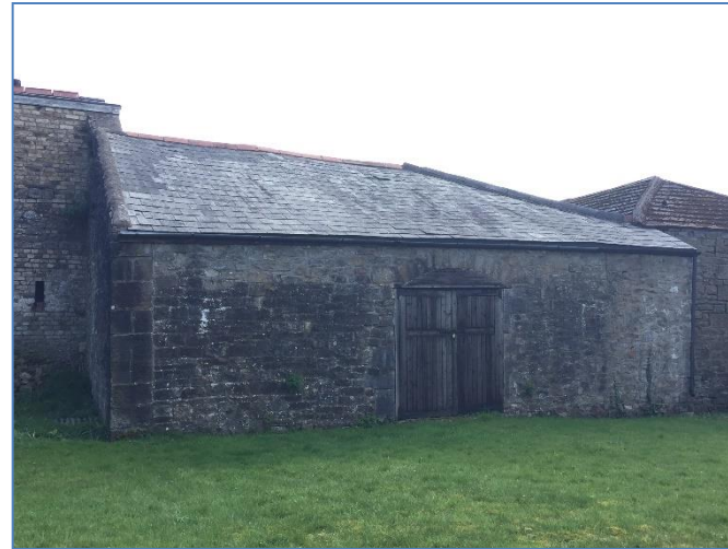
Photograph 18. Building D. The western elevation.
