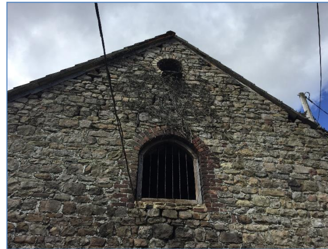
Photograph 4. Building B, eastern section. The eastern elevation with gappy verges.
