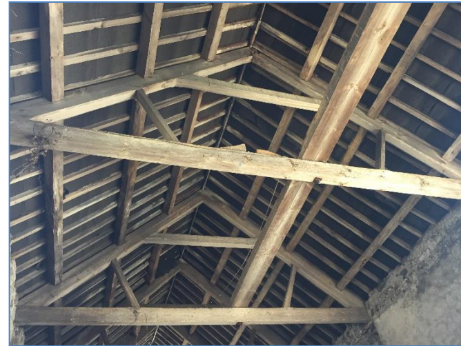
Photograph 6. Building B, eastern section. The tie and collar beam roof construction.
