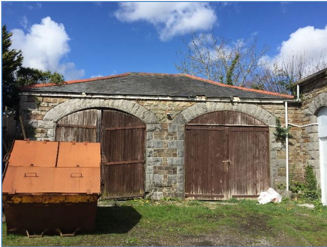
Photograph 21. Building E. The eastern elevation.
