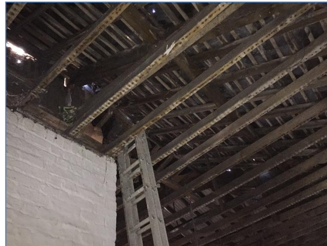
Photograph 20. Building D. The roof structure of the workshop, which has some sections of bitumen felt.
