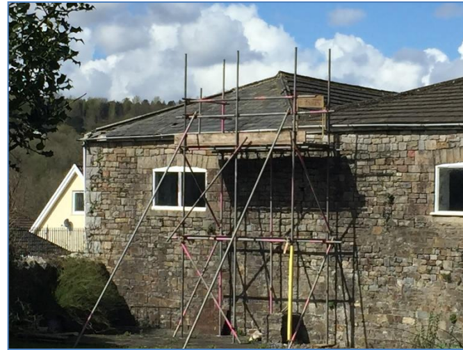
Photograph 26. Building F. The eastern elevation.
