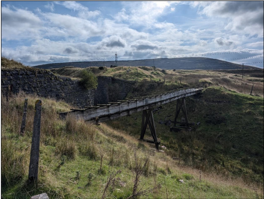
Plate 1. Relocated Listed Aqueduct (LB14143) view to south-east towards OB3
