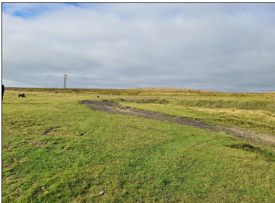
Plate 7. Rhas Las Dam (GM624), view to the west towards OB1 and OB2
