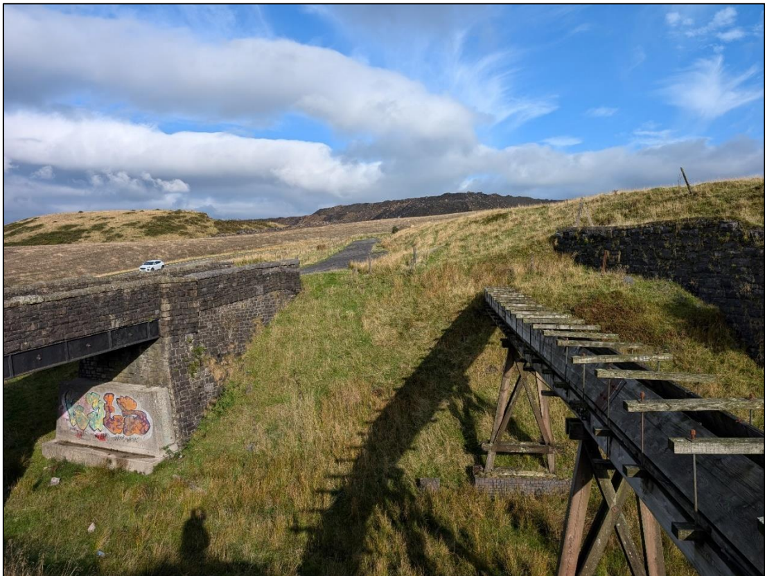
Plate 2. Relocated Listed Aqueduct (LB14143) view to the north towards the extraction area
