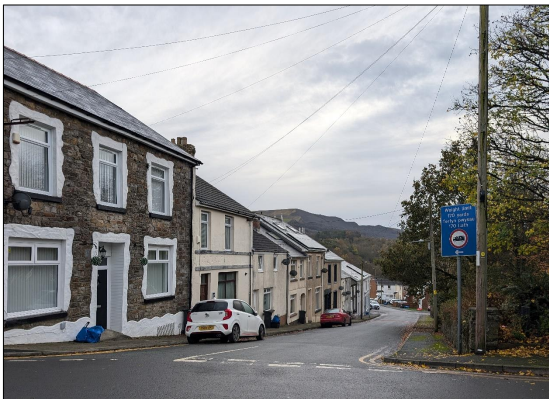
Plate 13. View south-east from Dowlais CA at the Dowlais Works Stables (LB 11478)
