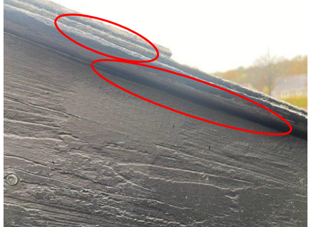
Photo 10: Example of Gaps Between Bargeboard and Roof Tiles on the Northern Elevation (Circled)
