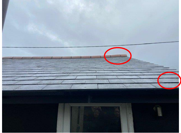
Photo 10: Example of Gaps Between Bargeboard and Roof Tiles on the Northern Elevation (Circled)
