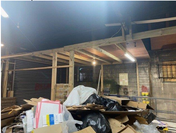
Photo 17: Timber Structure in Main Section of Workshop
