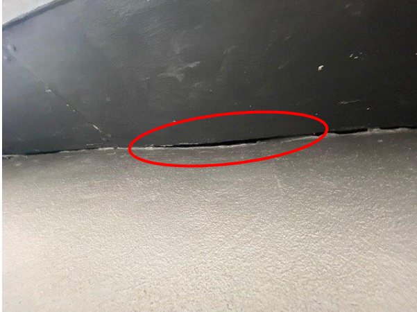
Photo 9: Example of Gaps Between Soffits and External Wall on All Elevations (Circled)
