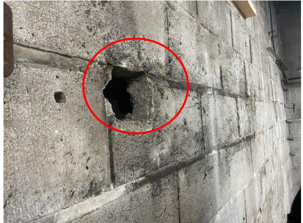
Photo 16: Hole in the Internal Breeze Block Walls Providing Access into the Wall Cavity (Circled)
