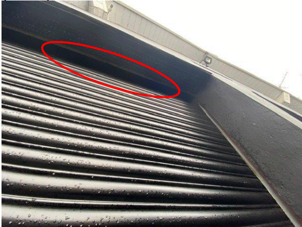
Photo 15: Gap Between the Metal Shutter Door and the External Wall on the Southern Elevation (Circled)
