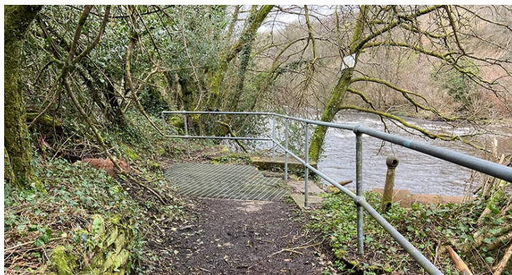
Figure 1-3 - Area of hard standing along the southern bank
