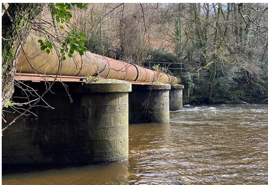
Figure 1-2: Existing Bridge Structure
