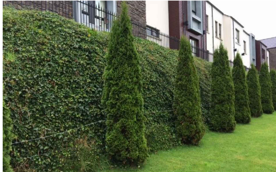
Retaining wall planted with ivy
