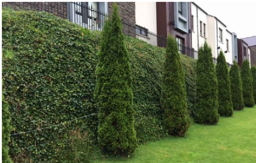
Retaining wall planted with ivy
