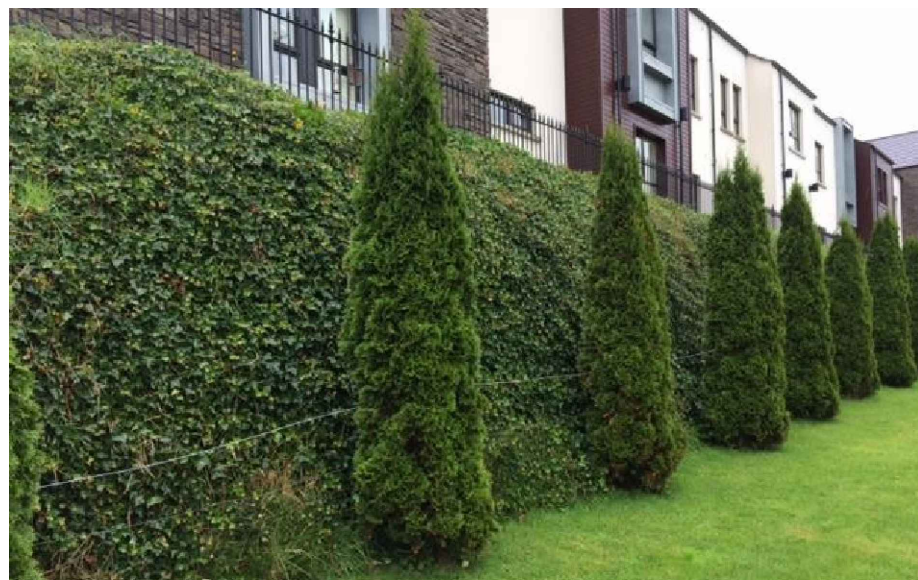
Retaining wall planted with ivy
