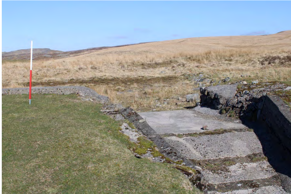
Photo 7: Concrete weir added to leat south of Pitwellt Pond
