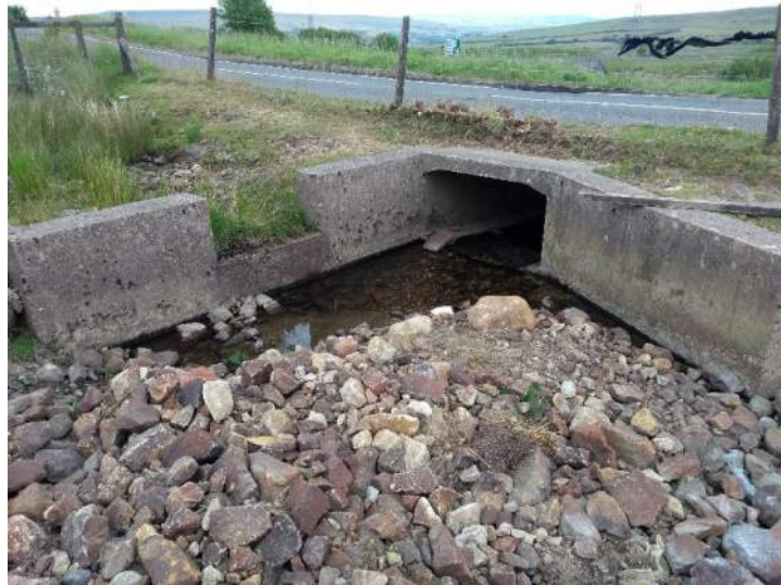
Photograph 3- Culverted stream at the southeast boundary of the Site.
