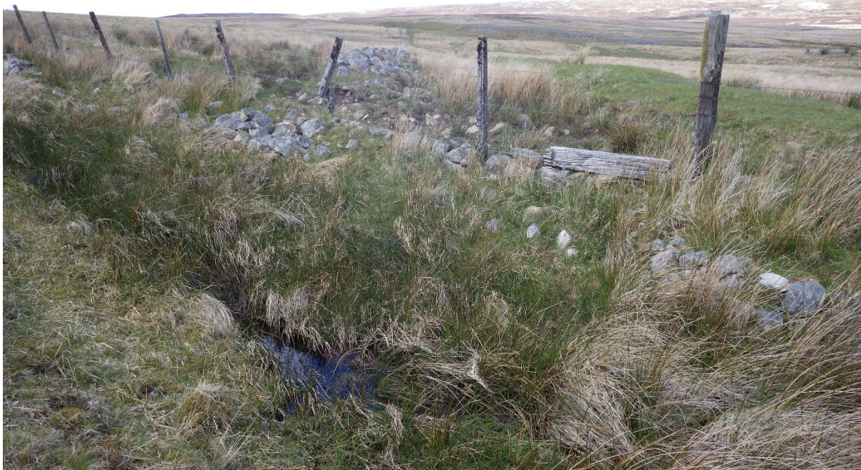
Photograph 20: View across Application Boundary to DCWW land showing perimeter drainage plus constructed bank and drainage channel within DCWW land. Looking N from NGR SO 0910 1065
