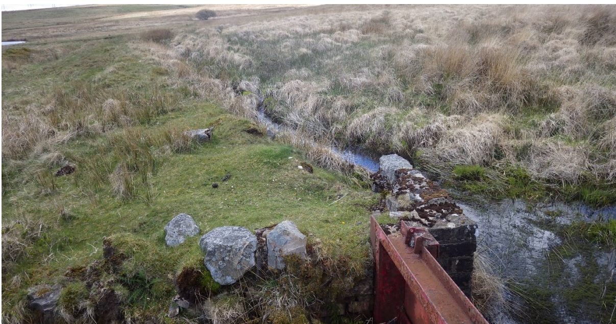
Photograph 4: Sluice gate and artificial channels near Jepson's Pond, looking W from NGR SO 0871 0931.
