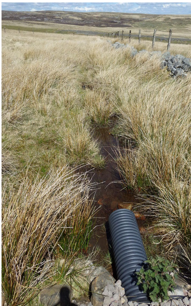
Photograph 21: Small pipe culvert installed at an access point. Looking NE from NGR SO 0886 1088.
