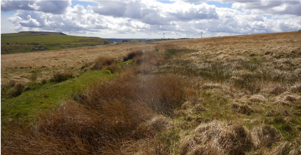
Photograph 5: Artificial drainage channel filled with rushes, looking WSW from NGR SO 0945 0958. The downslope bund has been breached in places, allowing water to flow downhill from the channel.
