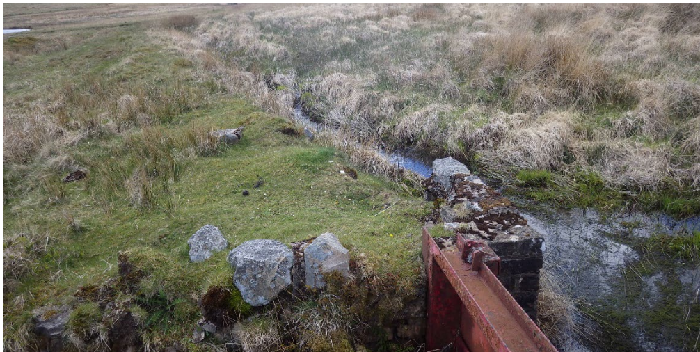
Photograph 6.7: An old sluice gate formerly used to control flows into Jepson's Pond. View NW, NGR SO 0872 0931.
