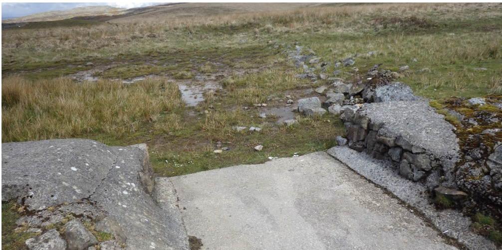
Photograph 6.5: Pitwellt Pond, showing the almost completely dry reservoir, with the constructed concrete outfall channel. View NW, NGR SO 0792 0969.
