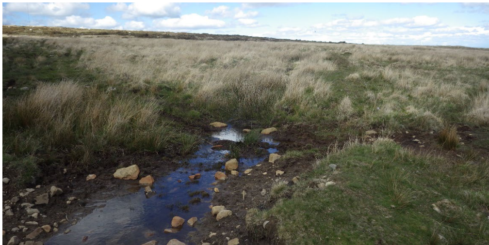
Photograph 6.8: Part of one of the cross-hill collector drains showing damage to the retaining bund as a result of livestock passage. View E, NGR SO 0871 0931.
