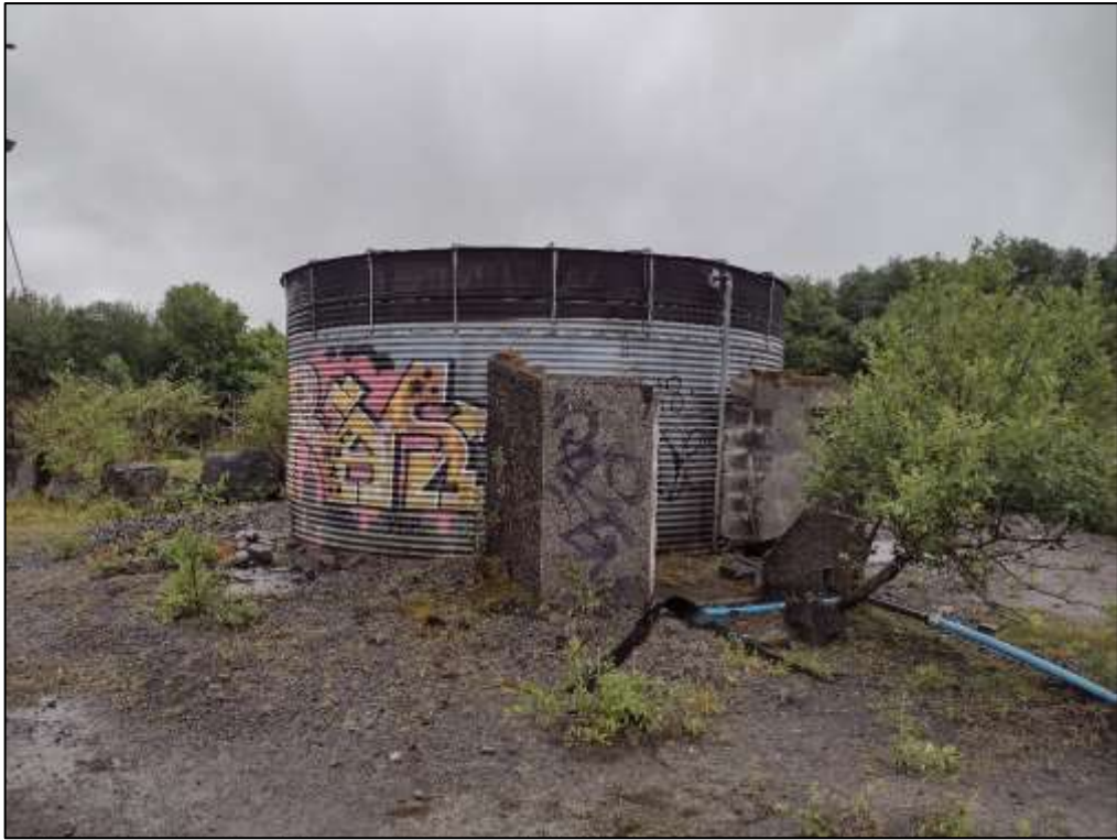
Photo 2. Storage tank, north facing elevation
