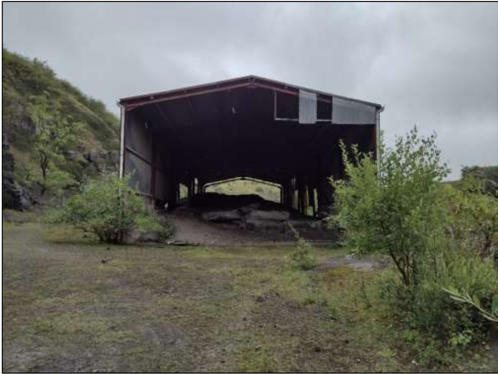
Photo 8. Storage building 1, south facing elevation
