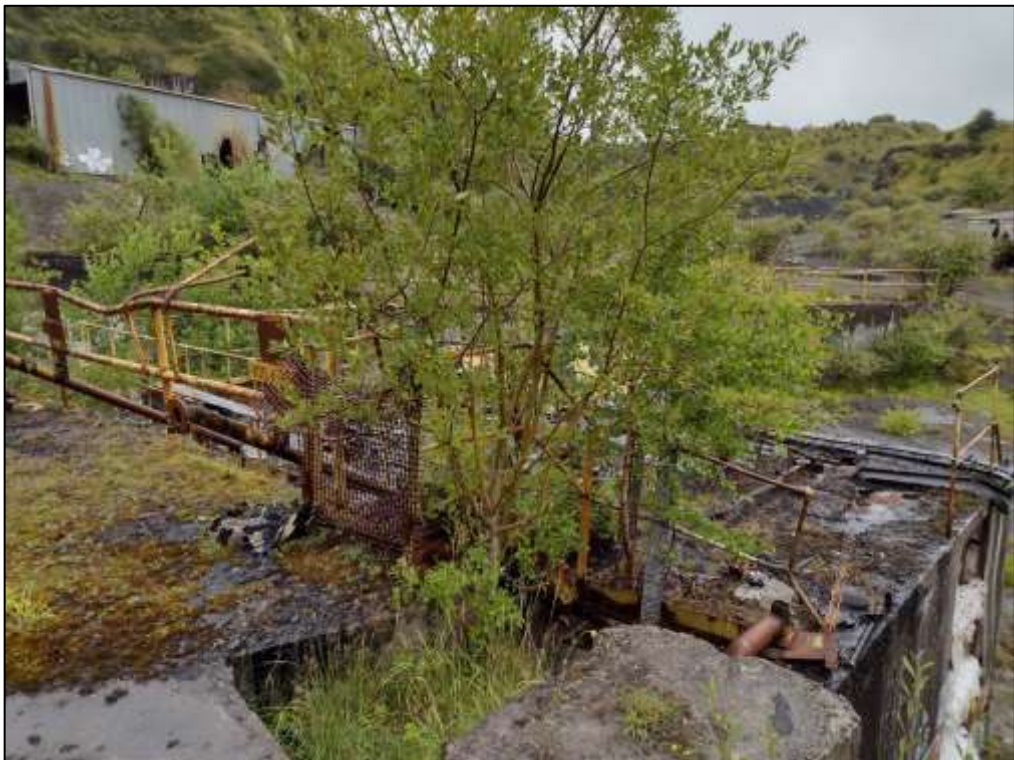
Photo 6. Remains of concrete structure 4 (Fig. 13, 6), looking north
