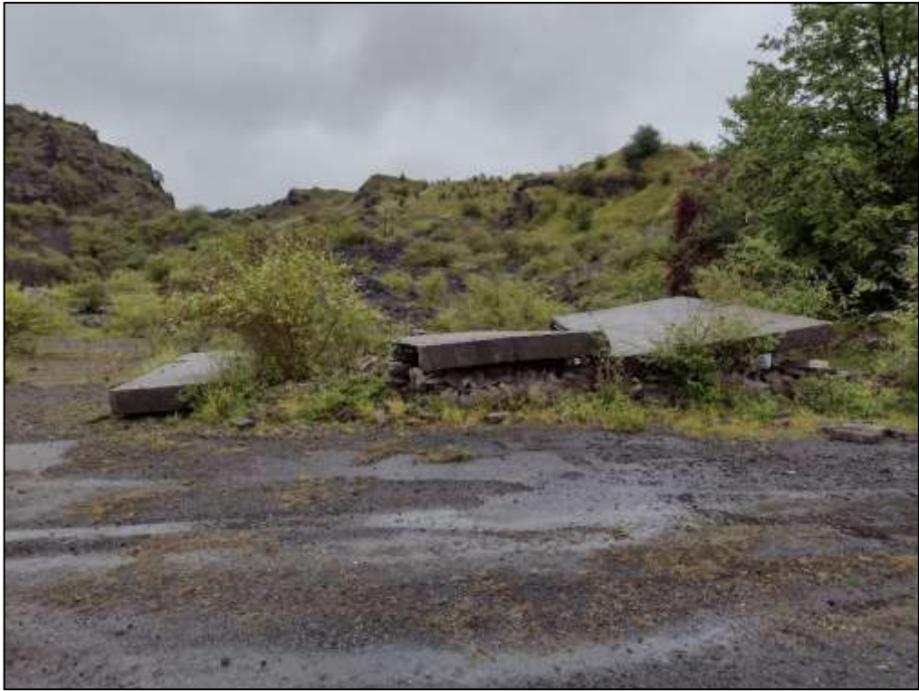
Photo 3. Remains of concrete structure 1 (Fig. 13, 3), looking north
