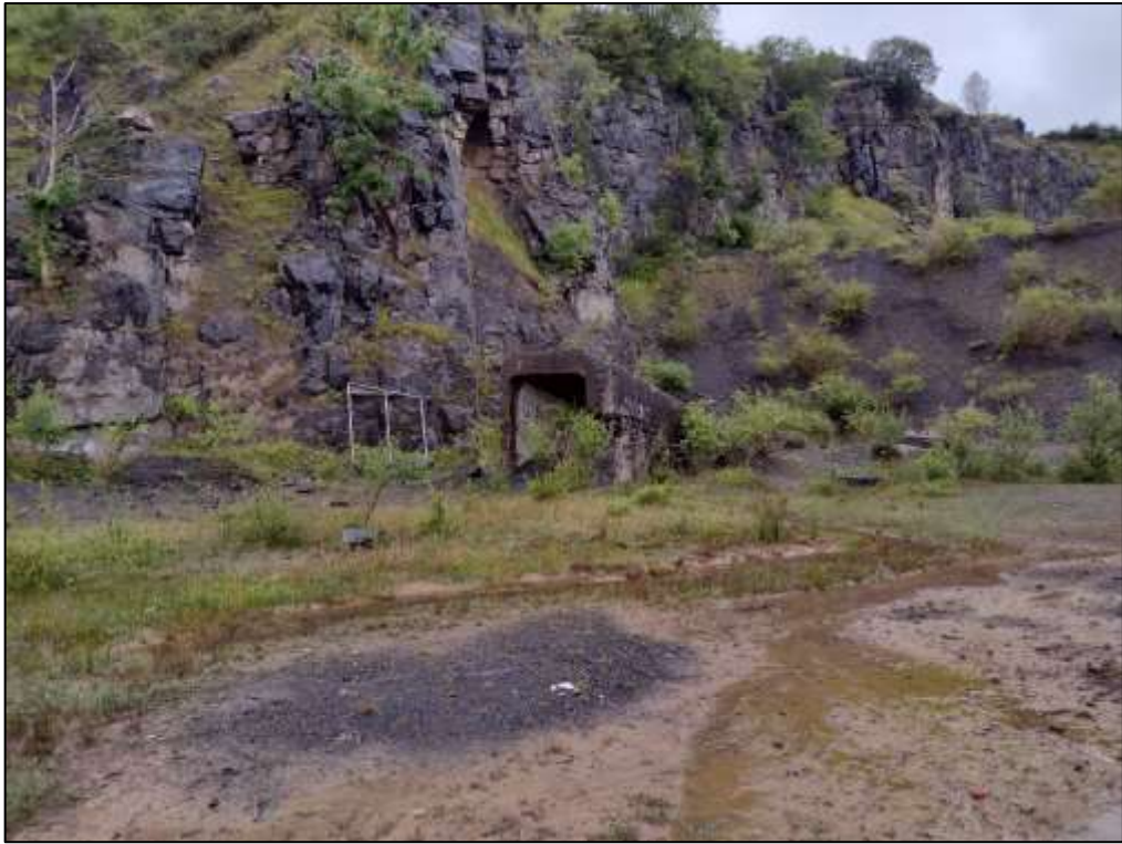
Photo 5. Remains of concrete structure 3 (Fig. 13, 5), looking north-west
