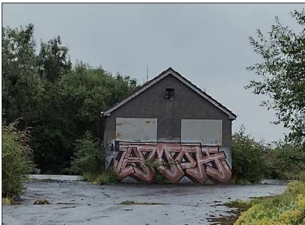
Photo 1. Weighbridge, west facing elevation
