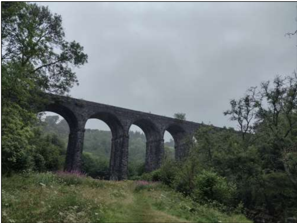
Photo 14. Pontsarn Railway Viaduct (Fig. 3, LB3) at base of valley, looking north
