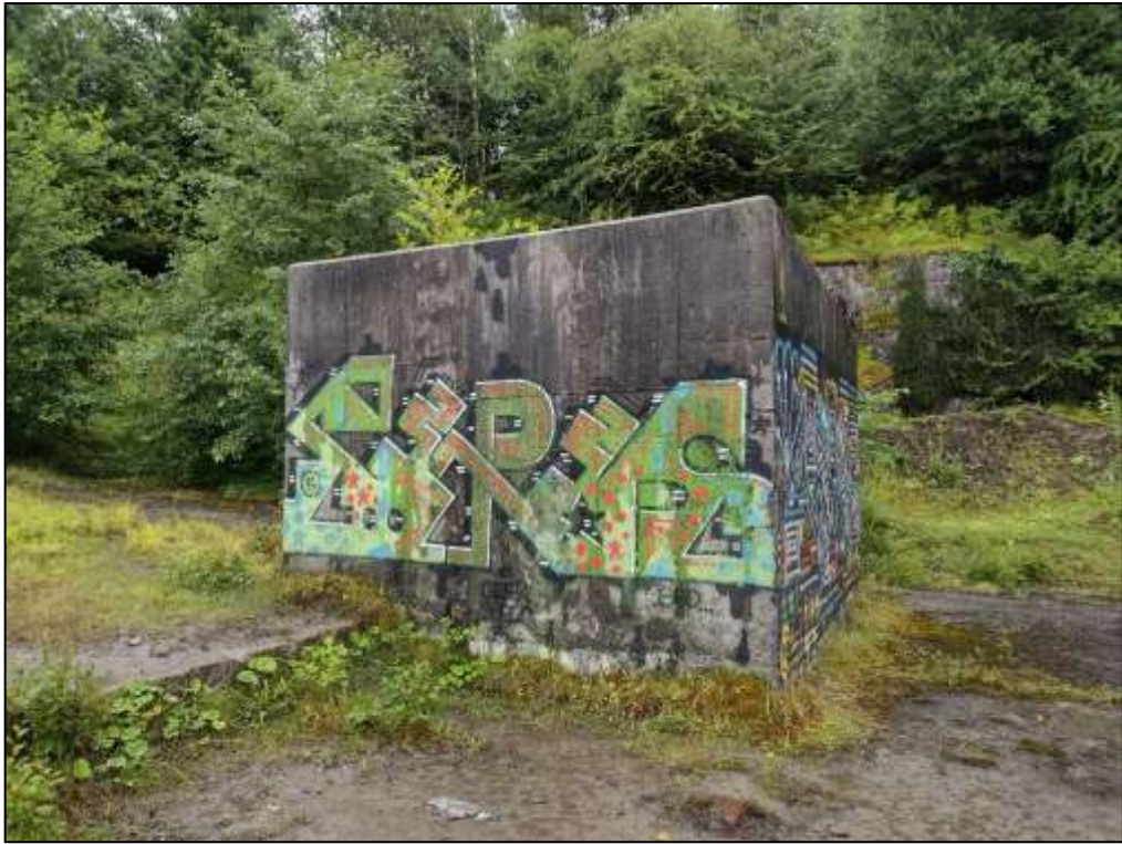
Photo 7. Remains of concrete structure 5 (Fig. 13, 7), north facing elevation
