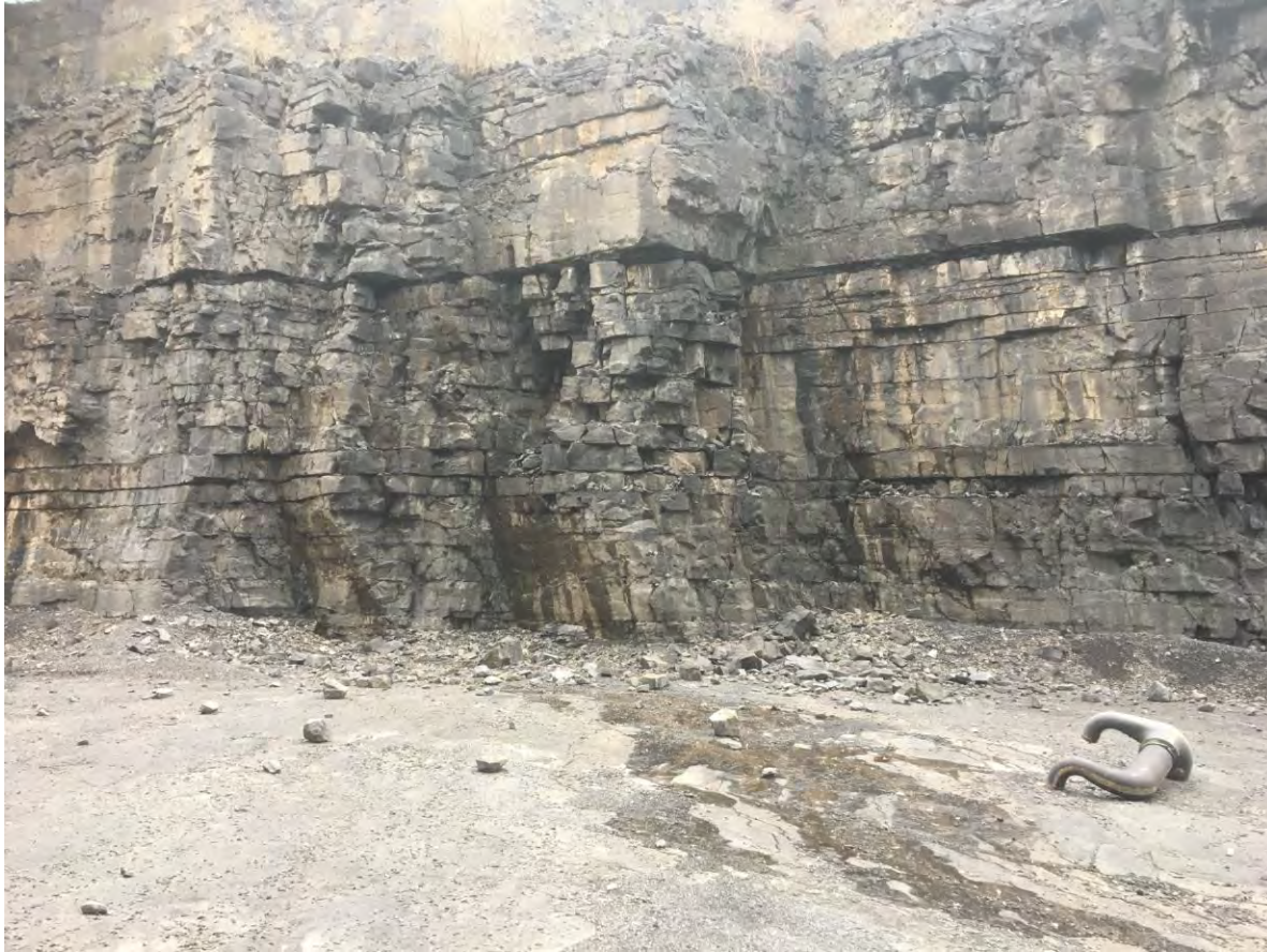
P009 – seepages and flow of water southwards along northern end of lower bench
