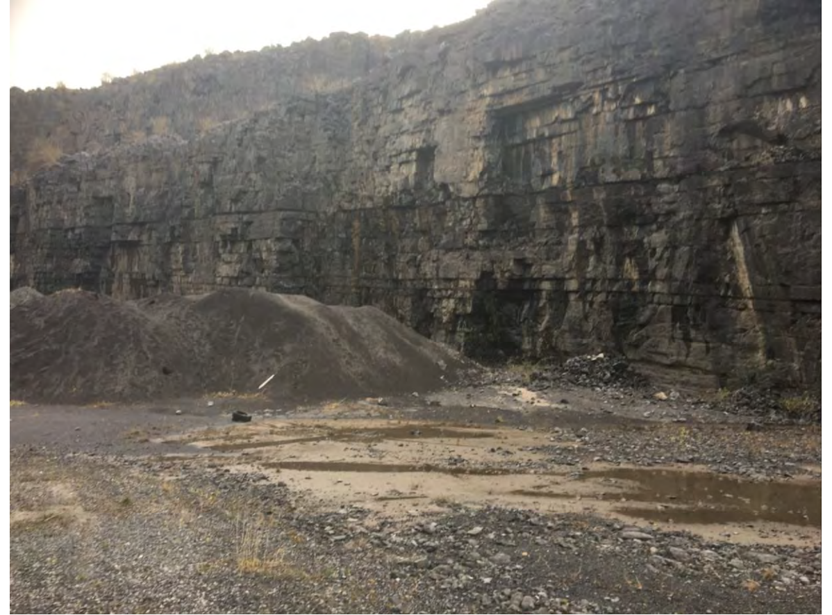
P002 - Seepages, many along bedding & standing water in S of Western arm
