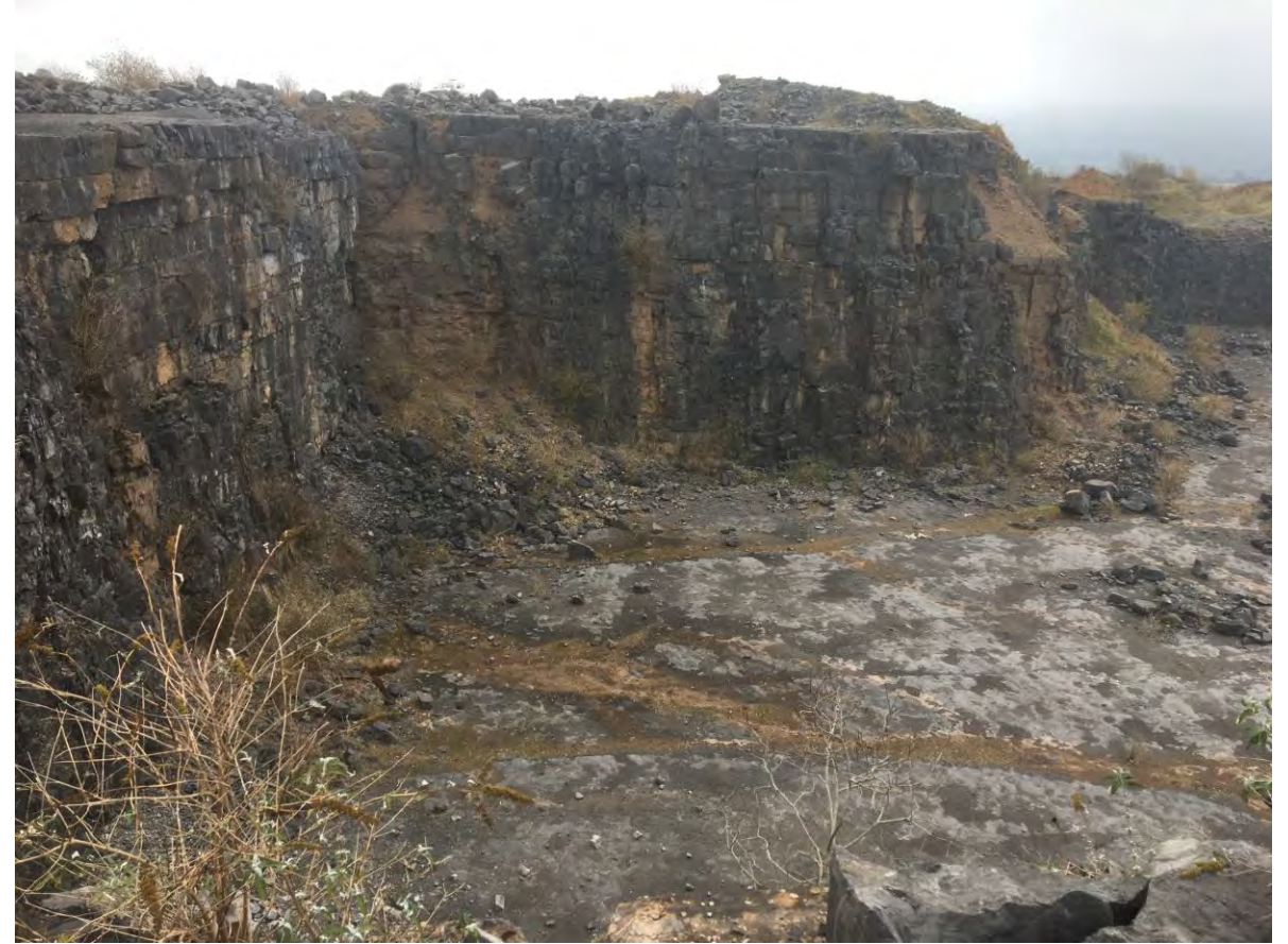
P018 – staining and algal growth marking flow of water from northern faces of western arm
