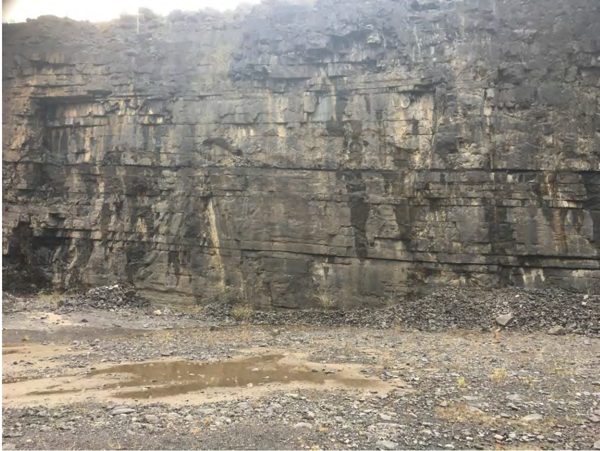
P001 – Seepages, many along bedding & standing water in S of Western arm
