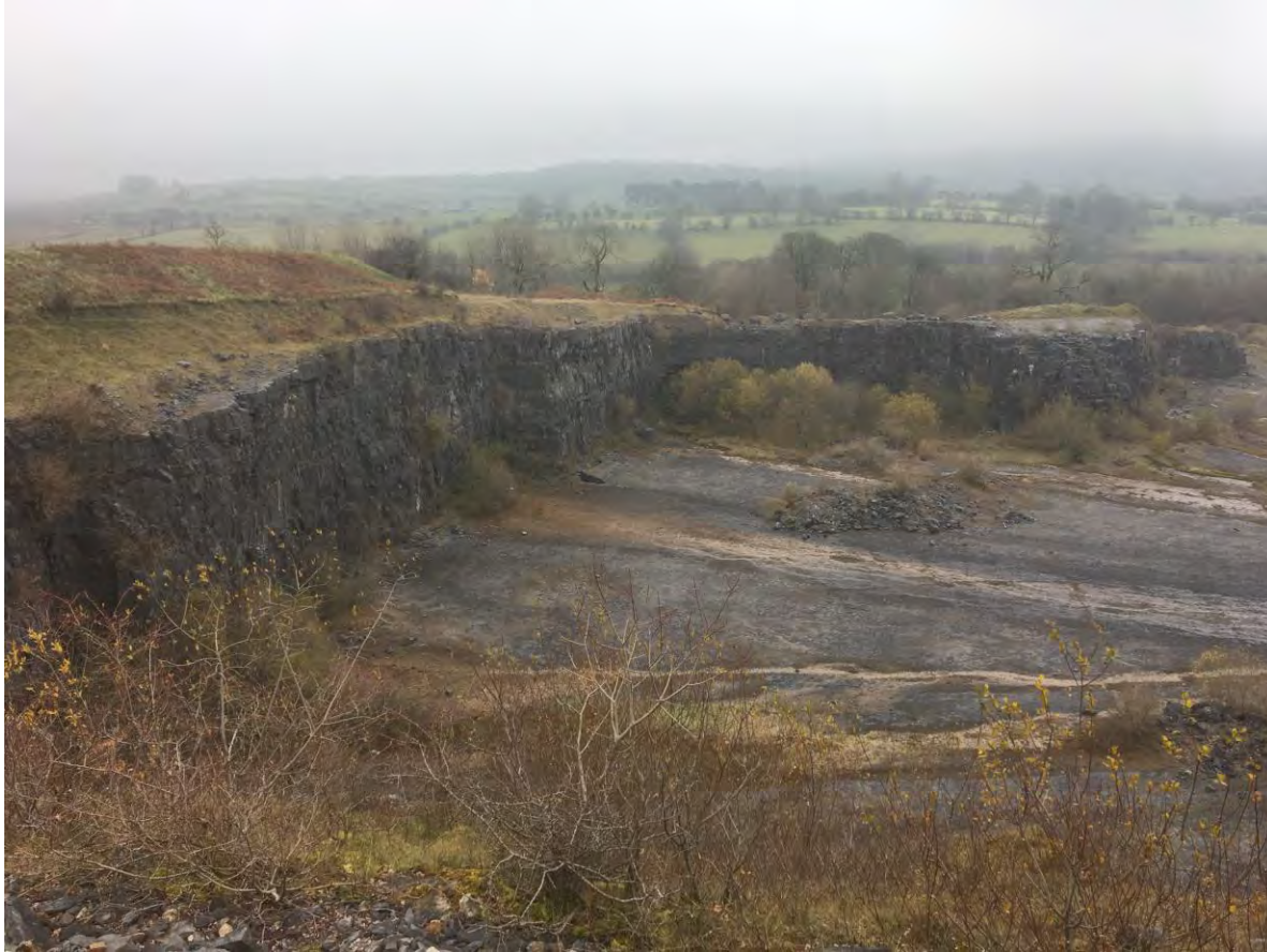
P030 – view of northern part of eastern arm looking east showing flow of water
