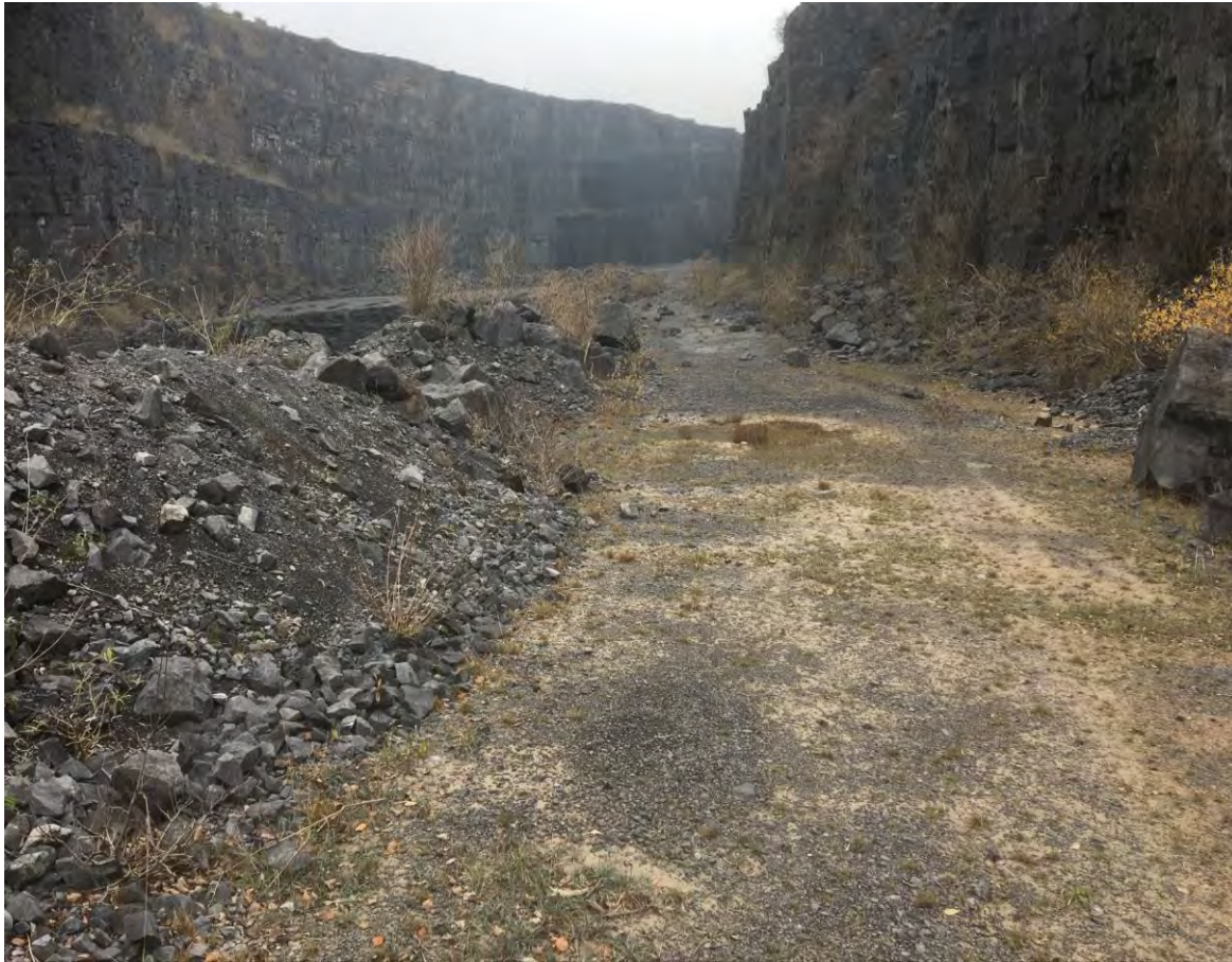
P029 – very limited ponding on benches
