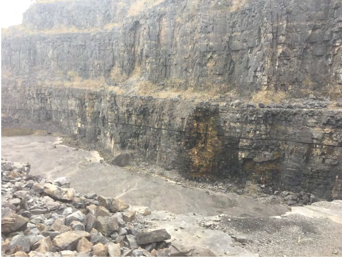
P027 – view of lower bench of western arm showing seepage as per P010
