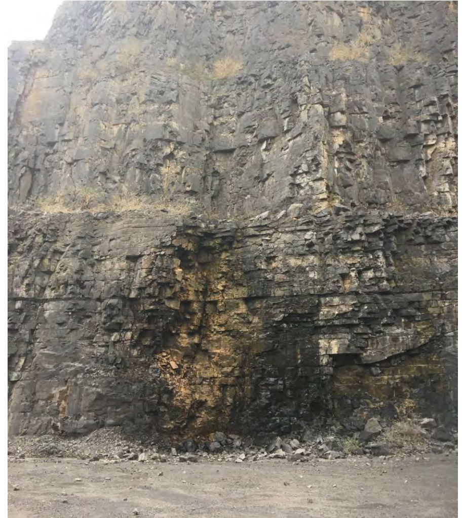
P010 – extensive seepage from fracture
