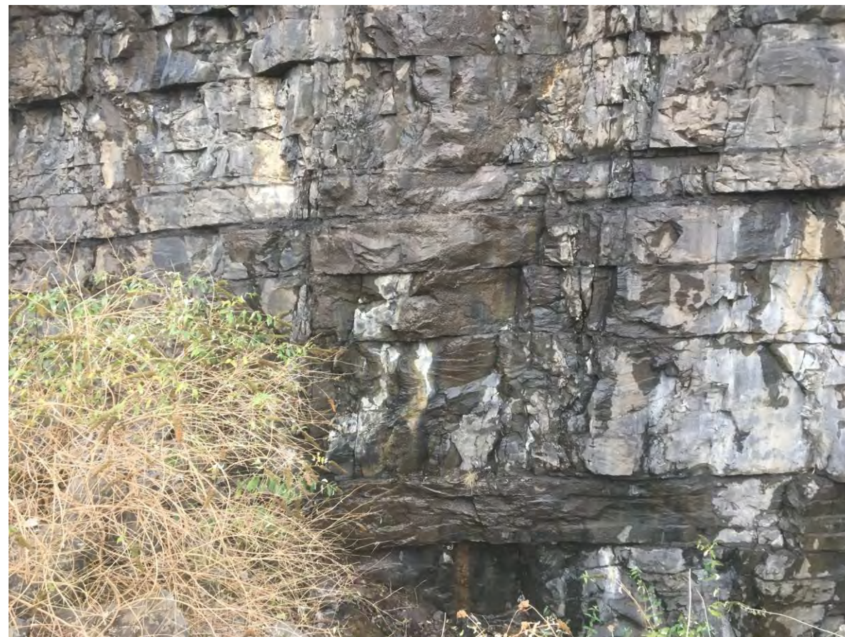
P047 – seepages in western face
