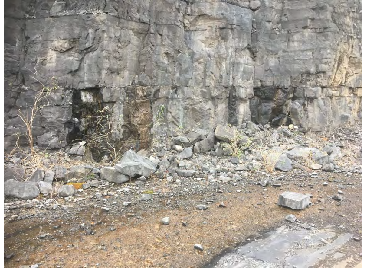
P063 – seepages along bedding planes
