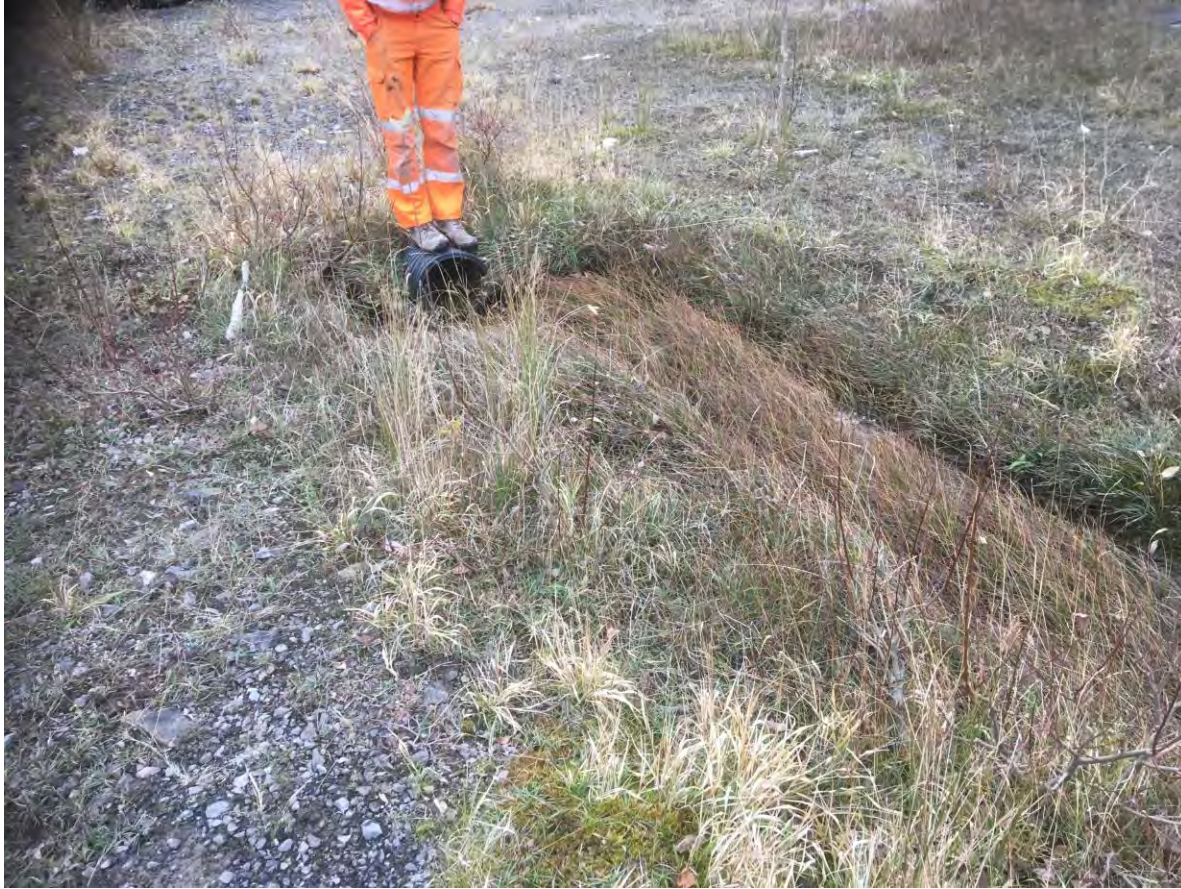
P086 – flow of water towards culvert
