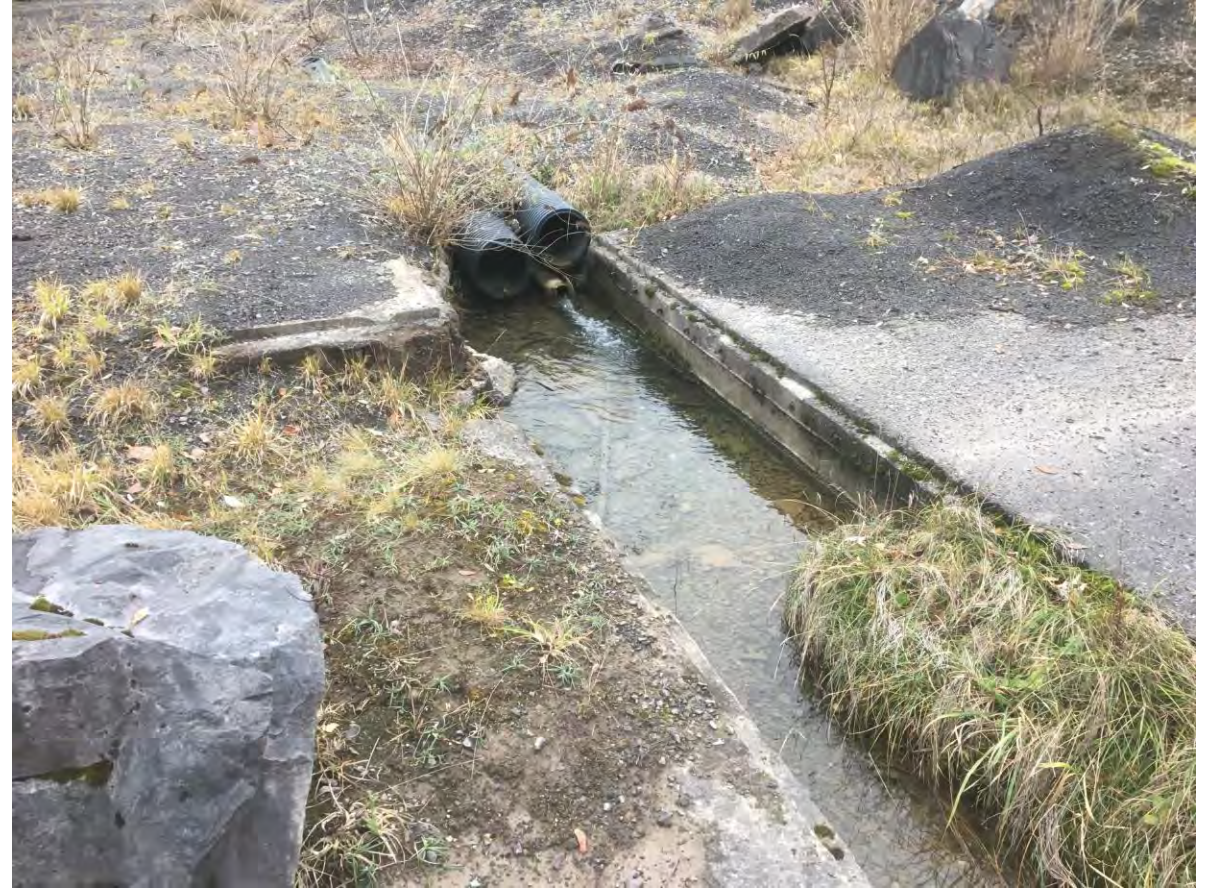
P085 – flow of water towards culvert
