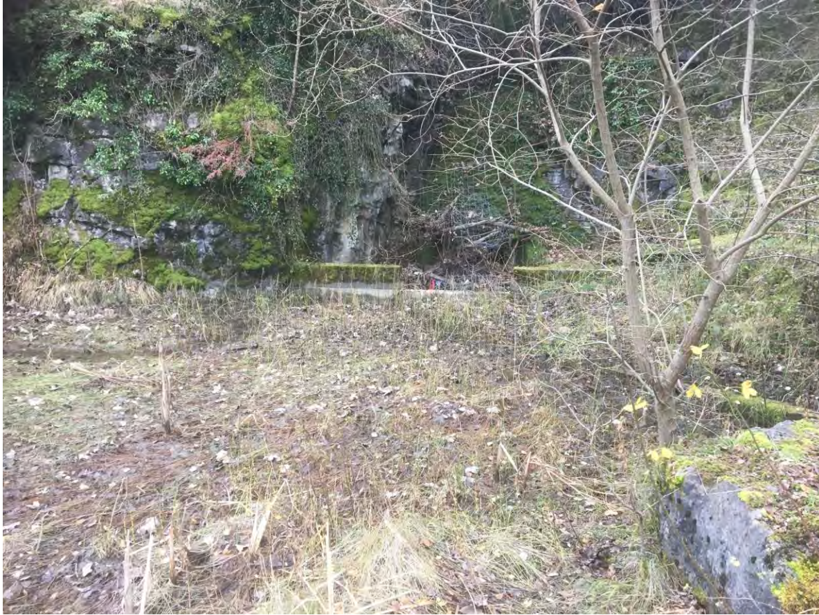
P084 – culvert in south
