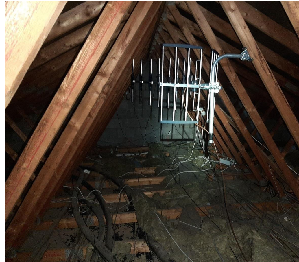
Photo 7. Club house building loft
