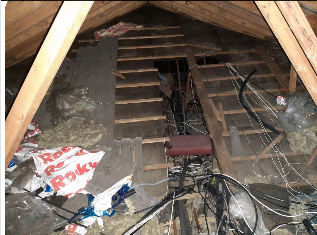
Photo 4. Club house building loft at hipped roof
