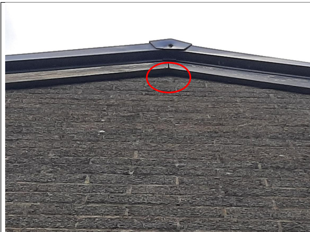
Photo 15. Changing room building suspected bat entrance
