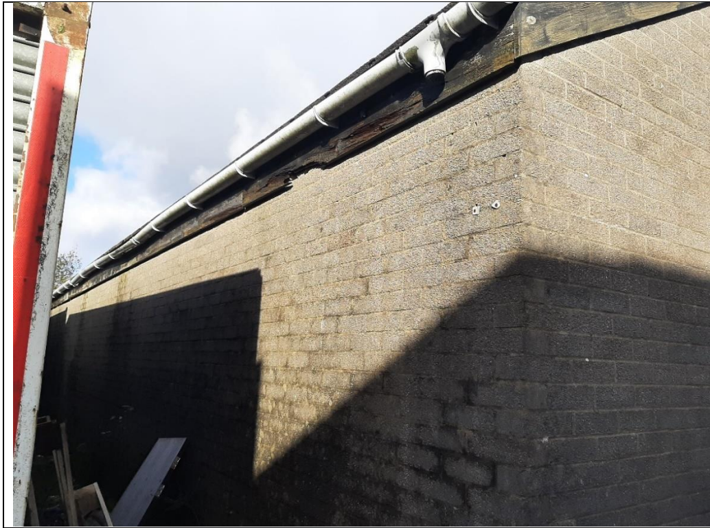
Photo 12. Changing room building rear
