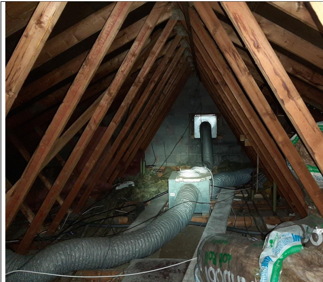
Photo 5. Club house building loft
