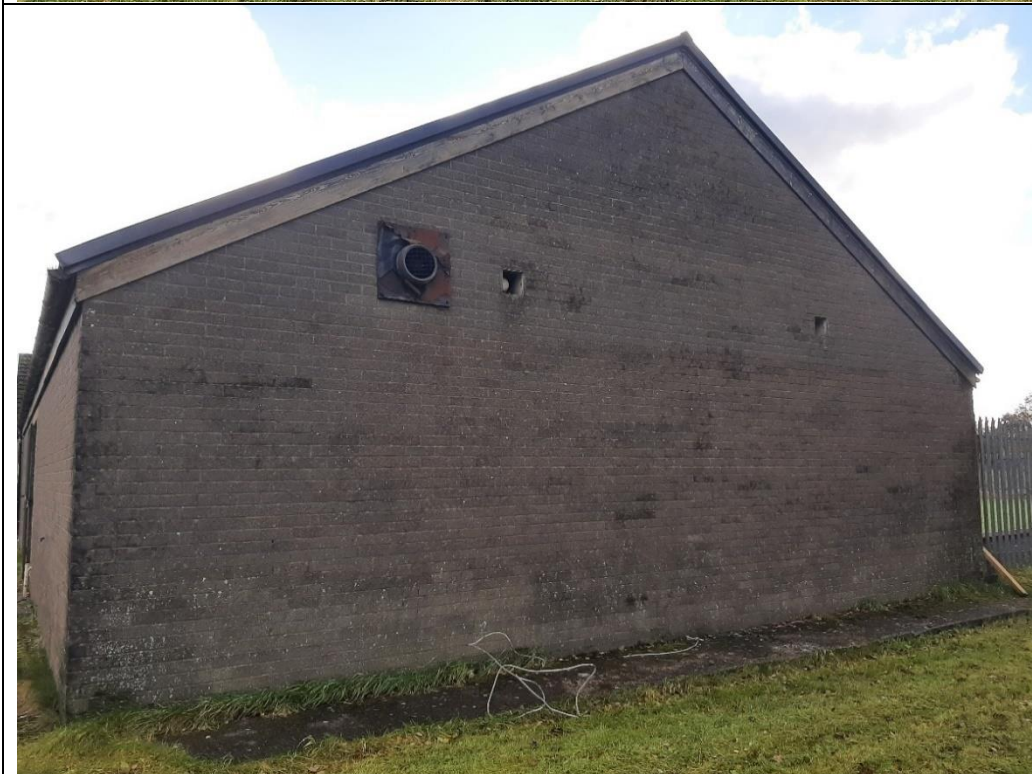
Photo 11. Changing room building northwest gable end
