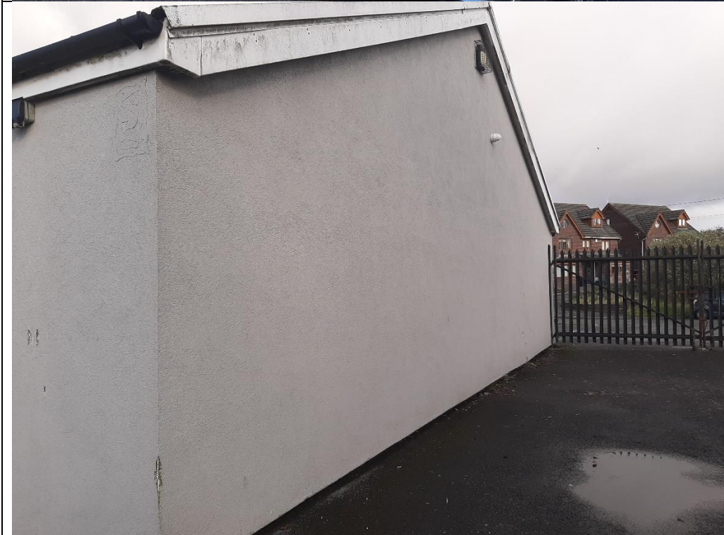
Photo 2. Club house building southeast gable
