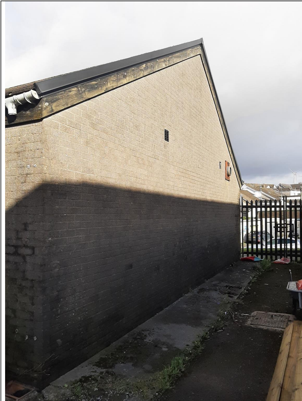
Photo 13. Changing room building southeast gable end
