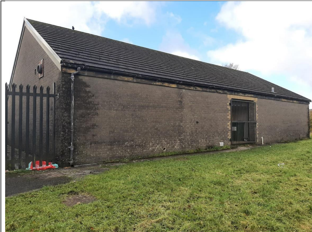
Photo 10. Changing room building front
