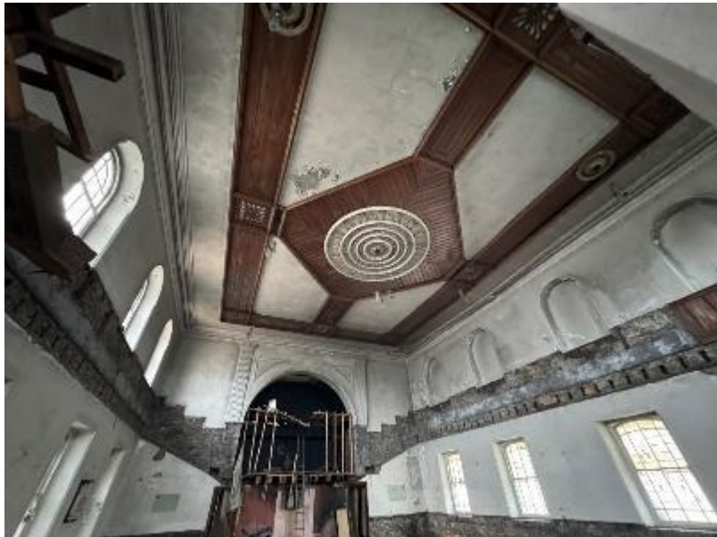
Photograph 19: Existing ceiling in the Main Chapel
