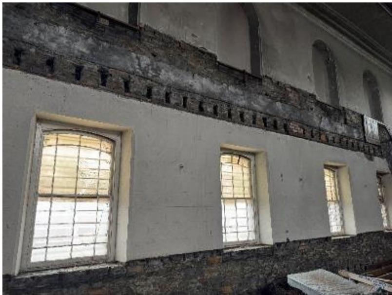
Photograph 10: Redundant wall pockets for the timber upper floor chapel seating
