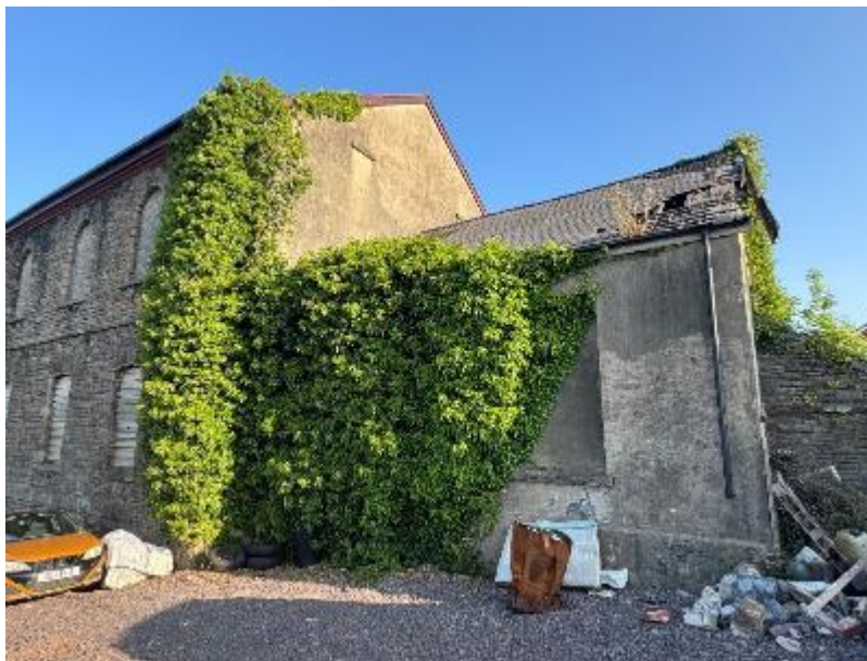
Photograph 5: Existing rear extensions (South Elevation)
