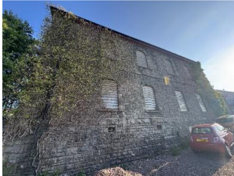
Photograph 26: Main Chapel (South Elevation)
