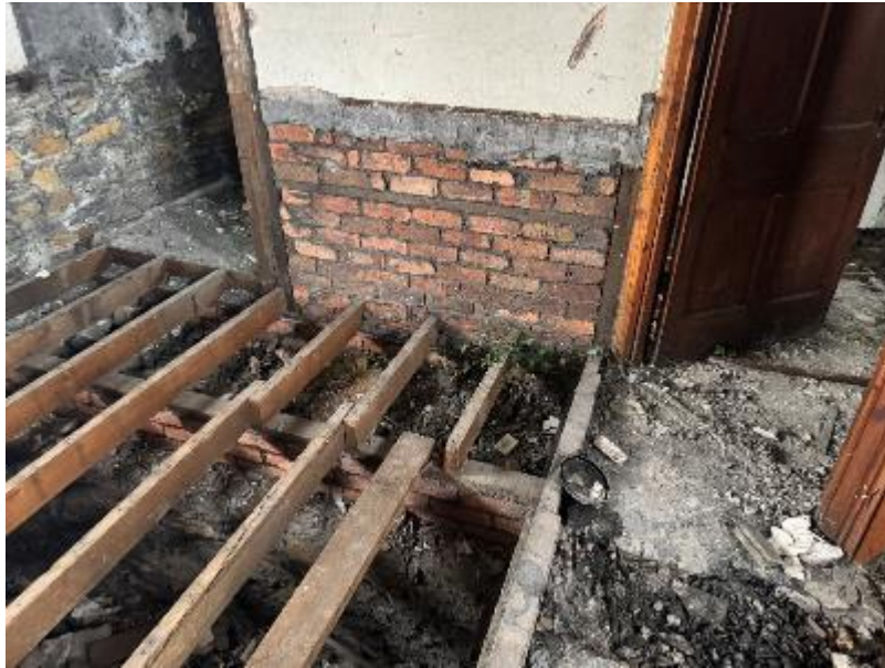
Photograph 14: Mainly suspended timber joisted floor on brick/stone sleeper walls
