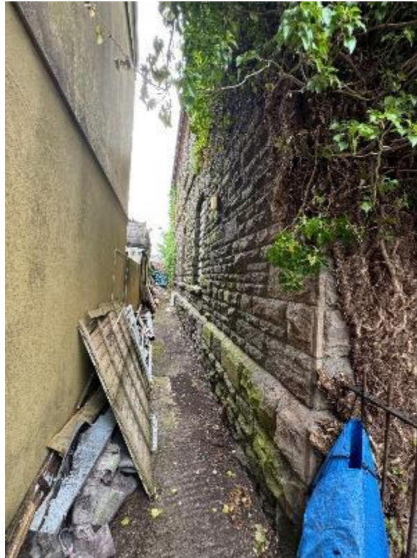
Photograph 3: North side elevation of the Main Chapel building
