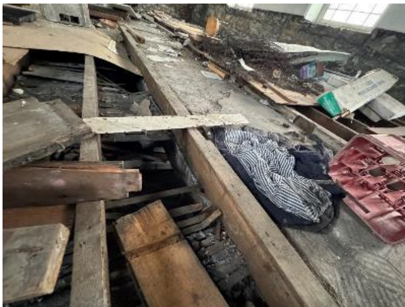
Photograph 25: Concrete slab spanning over the basement walls
