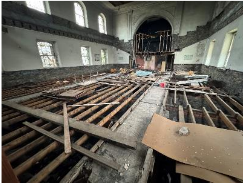
Photograph 9: Main Chapel (General View – looking East)
