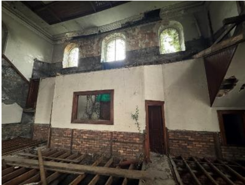
Photograph 22: Brickwork separating wall between the Main Chapel / Entrance Lobby
