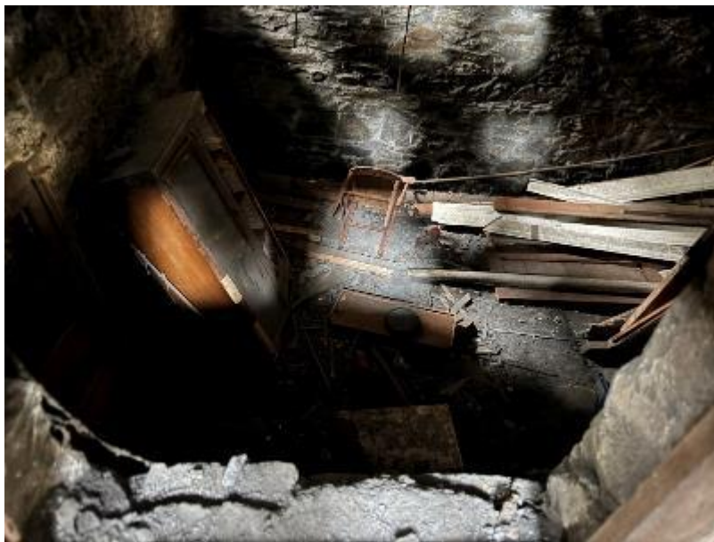
Photograph 23: Partial basement beneath the Main Chapel
