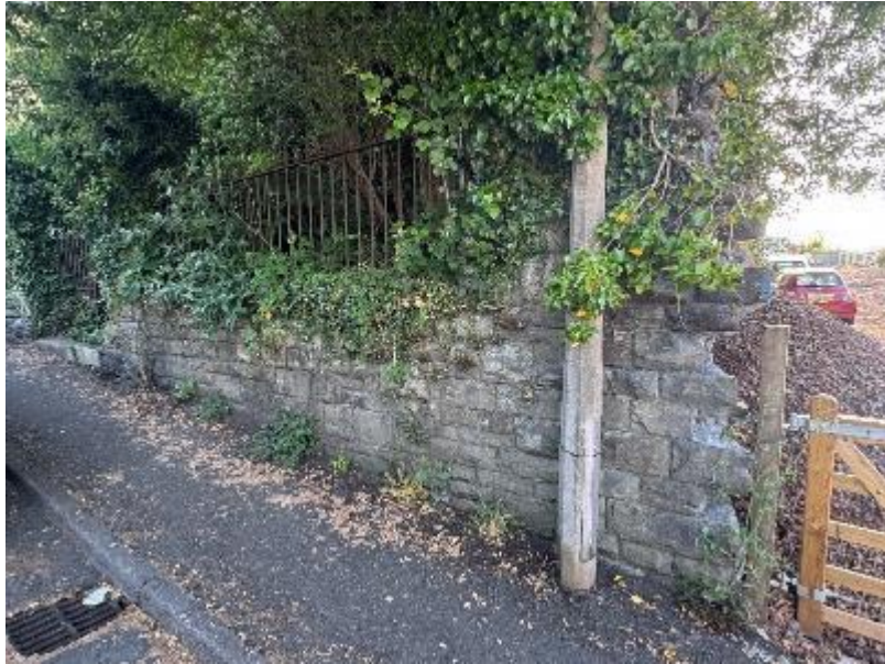
Photograph 28: Low-level boundary wall to the front elevation
