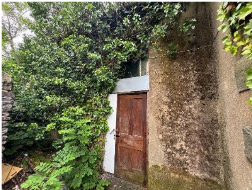
Photograph 4: Existing entrance door into the rear extension and Main Chapel
