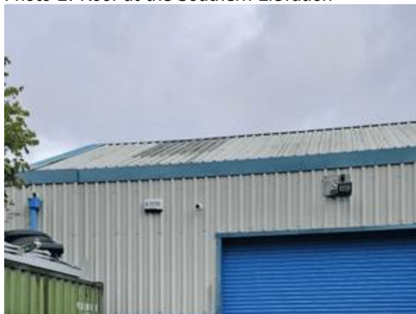
Photo 2: Roof at the Southern Elevation
