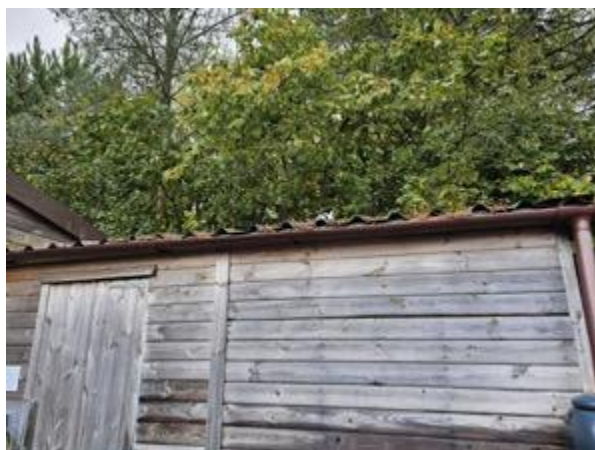
Photo 9: Roof at the North-Western Elevation
