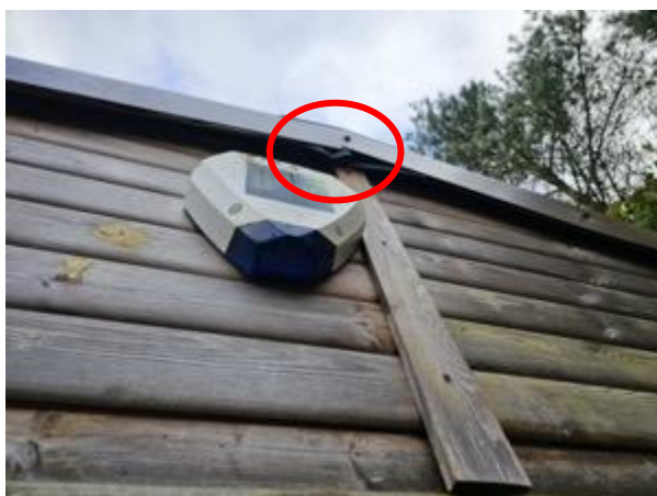
Photo 10: Gap Underneath the Metal Trim at the Apex (Circled)
