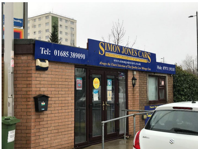
Photograph 3: Northern aspect of B2.
