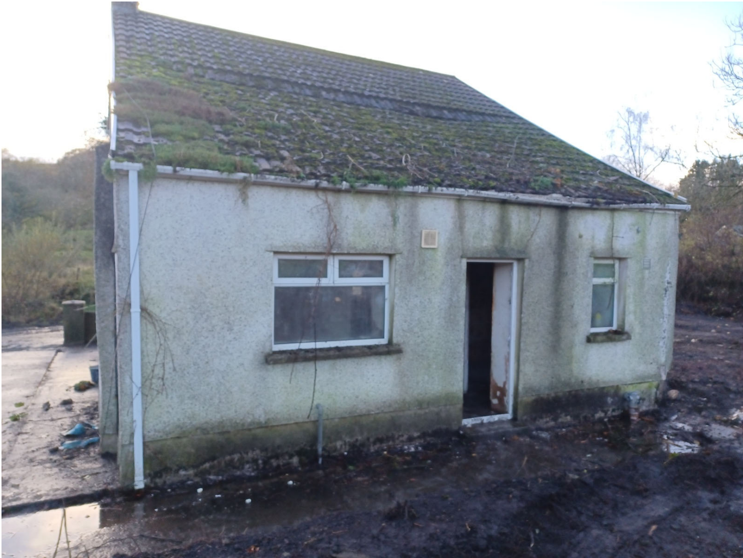
Photo 6 – Rear of House prior to renovation
