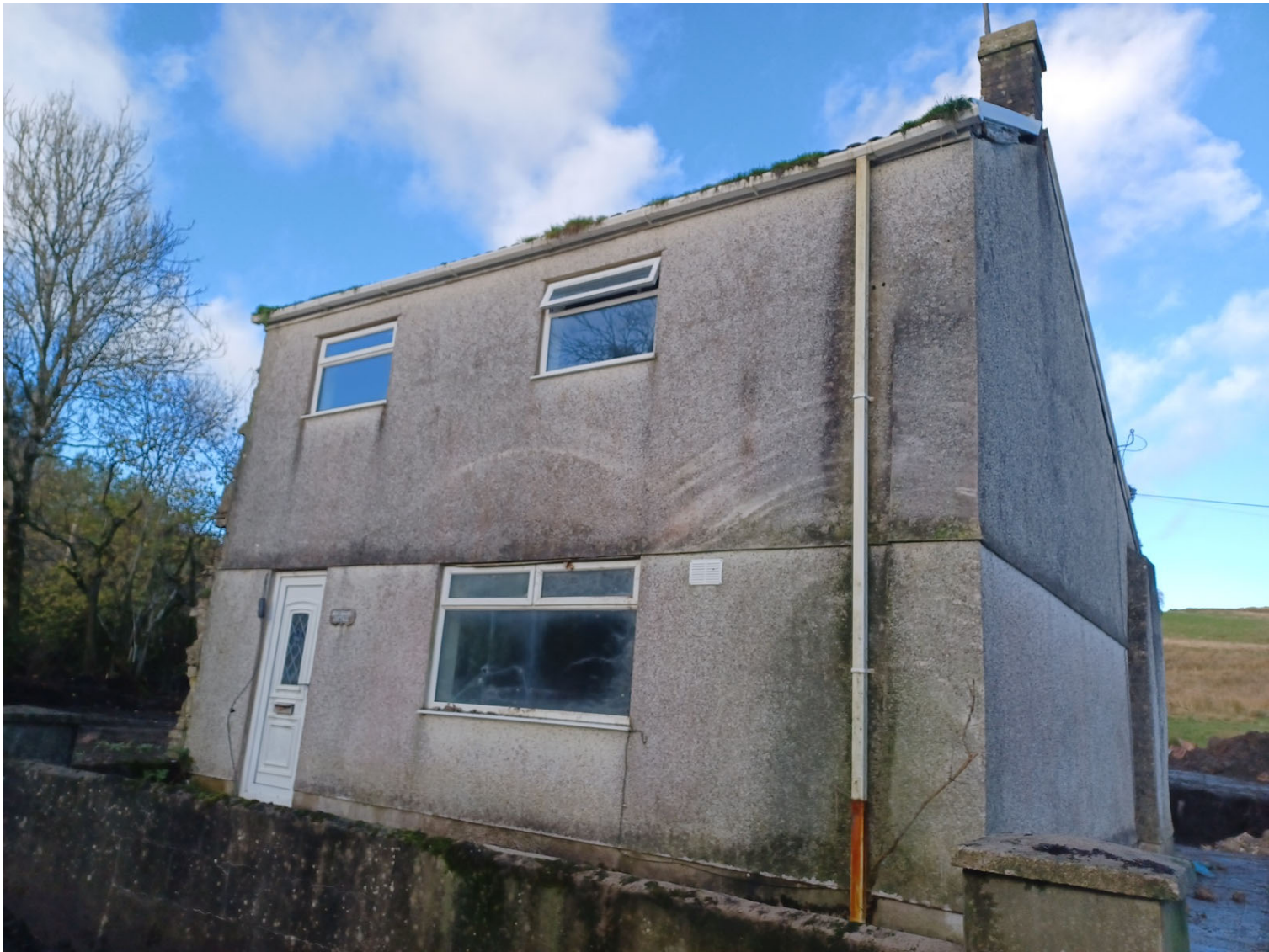
Photo 5 – Front of House prior to renovation
