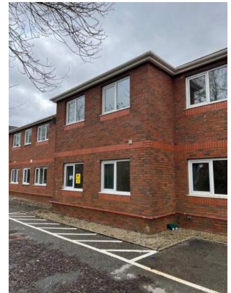
Carbon Steel LP Gas Pipe (East Elevation)
