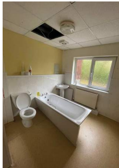
Existing Bathroom (Bathroom 1 / G032)
