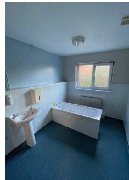
Existing Bathroom (Bathroom 1st / F104)
