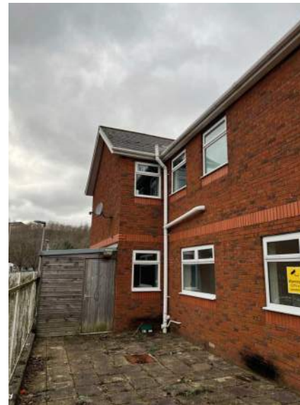
Rear of Extension (South Elevation)
