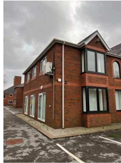
Corner of Community Hub (North/East Elevation)
