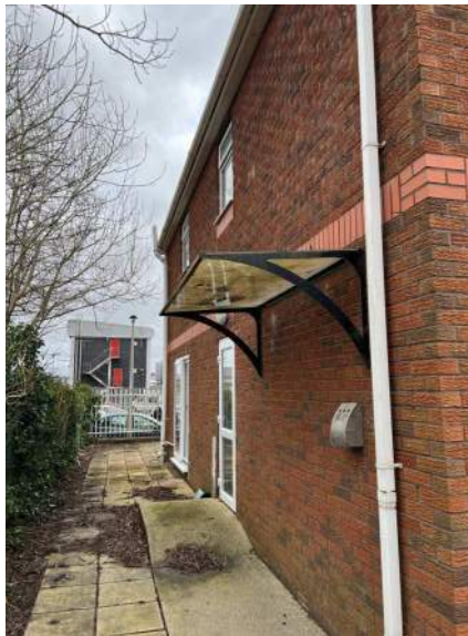
Access & Escape Doors, ESA (East Elevation)
