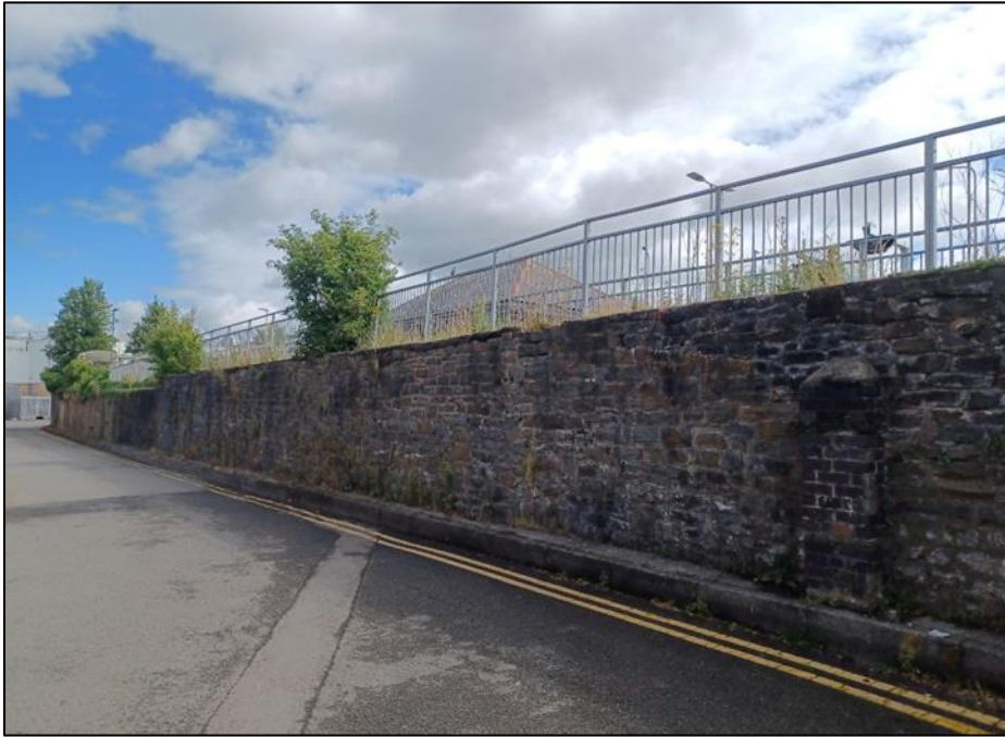
Photograph 4: Retaining wall on site where sand martins were confirmed breeding.
