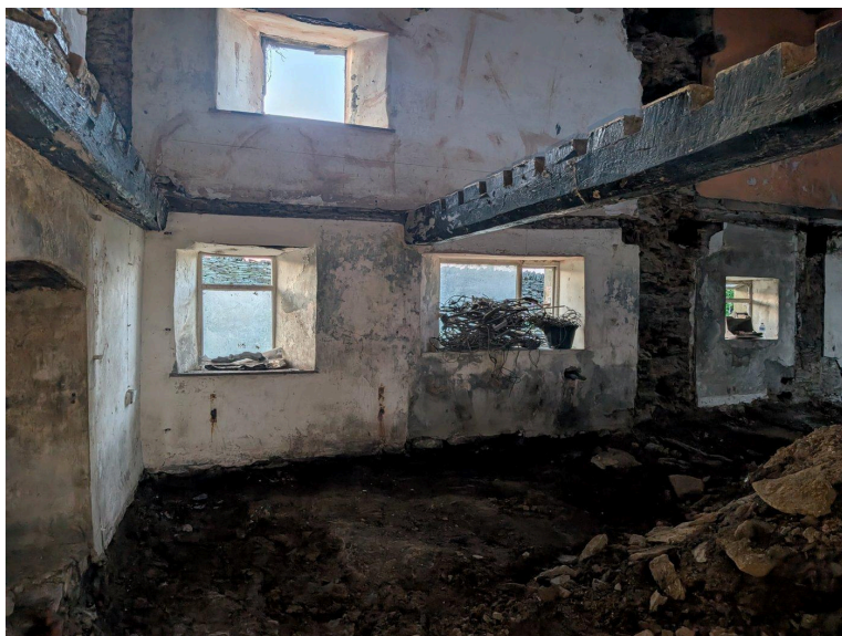
Plate 5 - Guttered ground-floor room showing multiple small window openings, exposed bressummer/ceiling beams and a bare earth and rubble floor.
