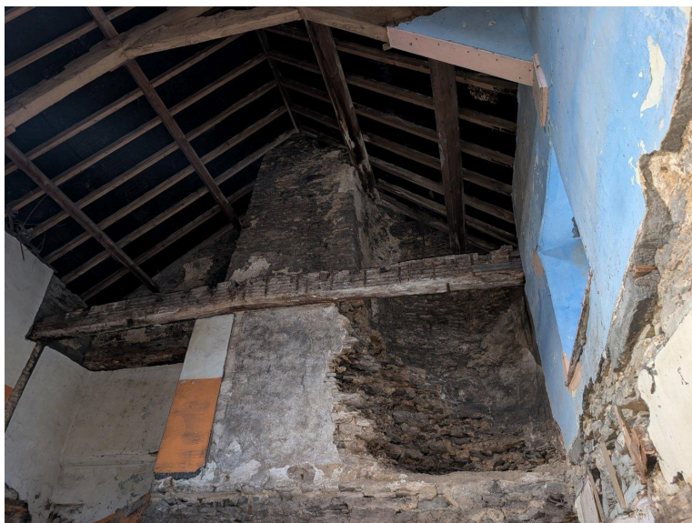
Plate 3 - Internal corner showing exposed roof timbers meeting a stone chimney breast,
