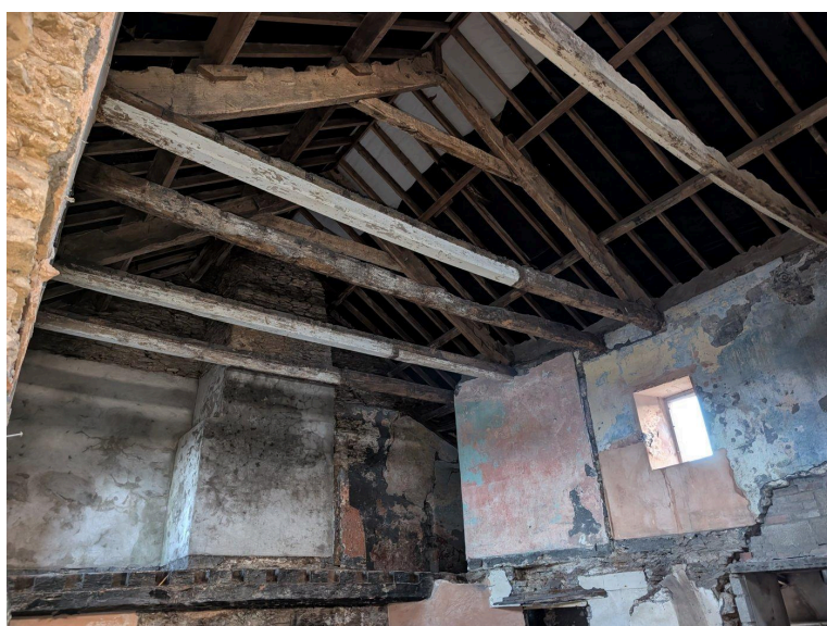
Plate 2 - Farmhouse roof structure viewed from below, showing exposed pitched roof timbers and rafters over degraded plaster and bare stone walls, with a small square window opening to the gable.
