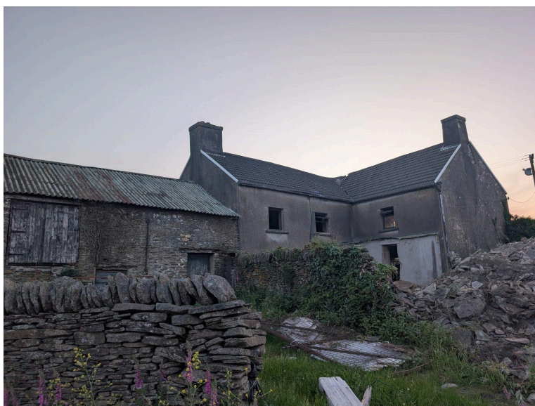
Plate 10 - Site context: the farmhouse and attached barn range viewed from the rear, showing tiled and corrugated roofs, chimney stack.
