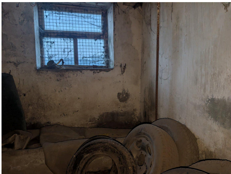
Plate 8 - Barn/store corner showing a mesh-covered window
