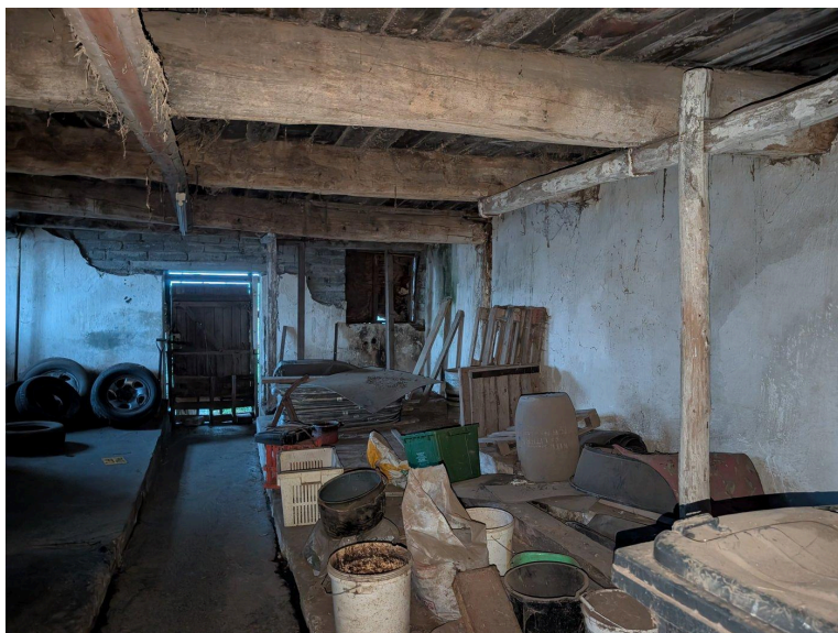
Plate 7 - Barn interior used for storage beneath exposed ceiling beams and timber roof structure, with an open doorway and stored materials
