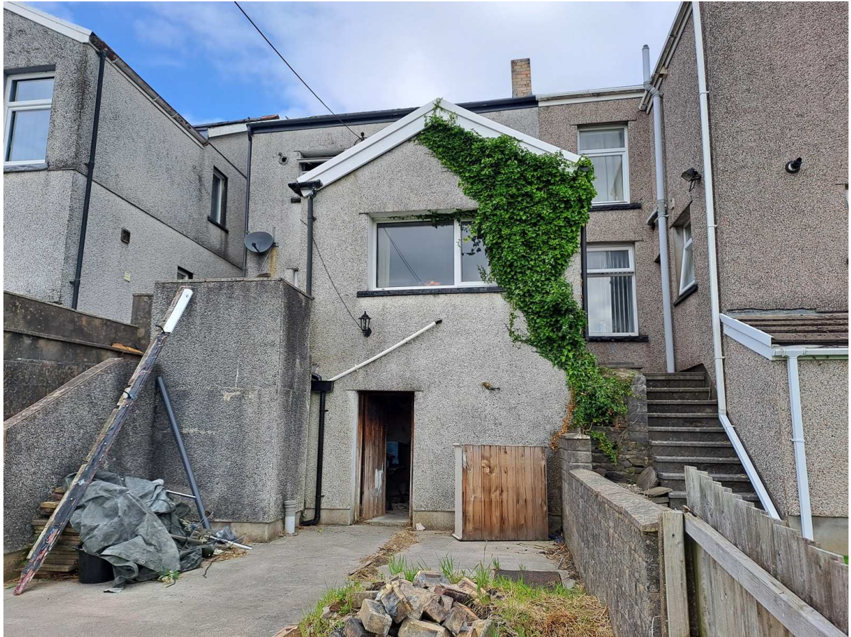
Photo 1 – Rear Elevation of Property
