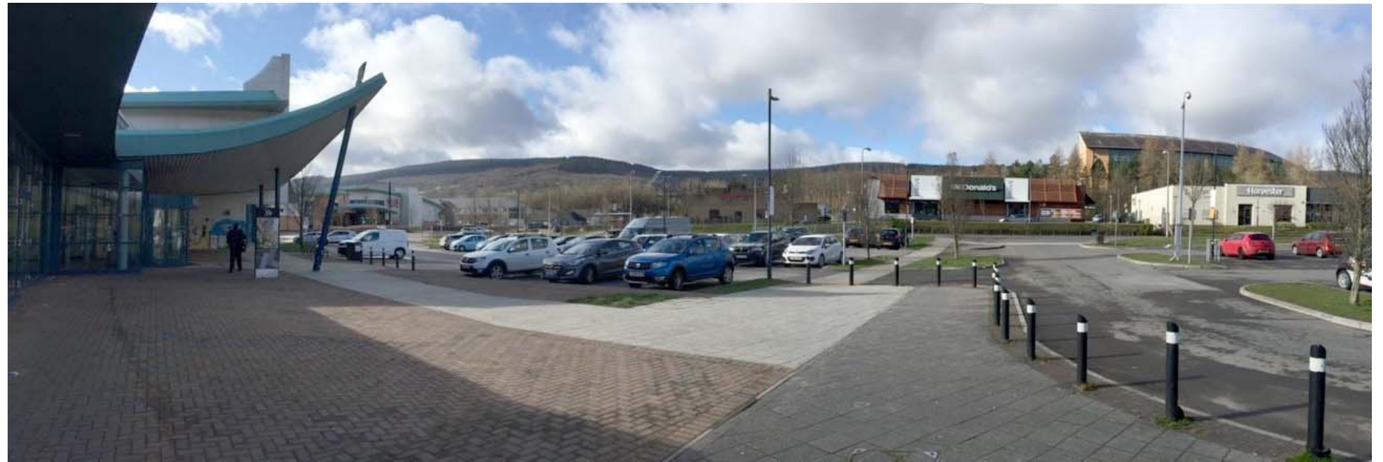
View of the Leisure Centre site and building entrance
