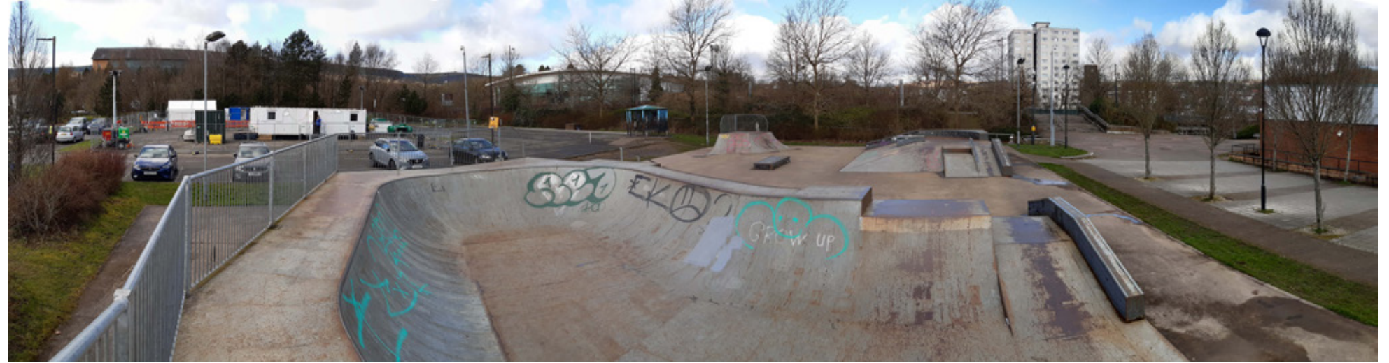
Existing Skate Park site view looking North
