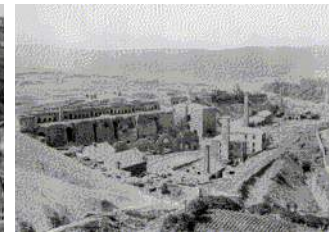
Penydarren Iron Works
