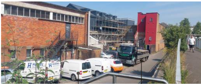
4 - Masonic Street from Platform
