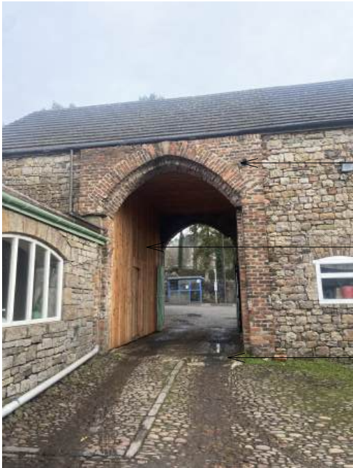
Existing entrance archway - view from courtyard
