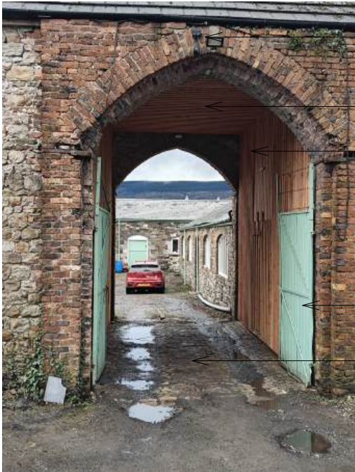
Existing entrance archway - view from Road
