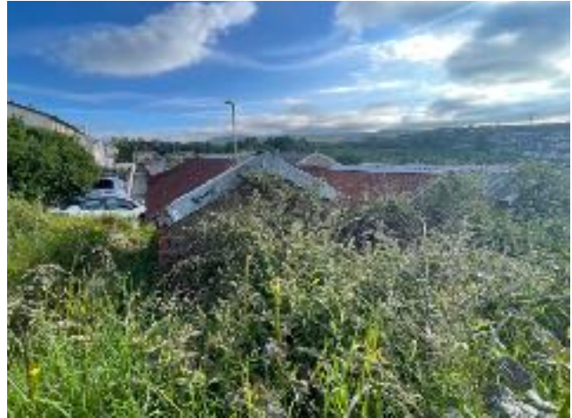
Photo 14. Garages within northeast corner of site view of roofs.
