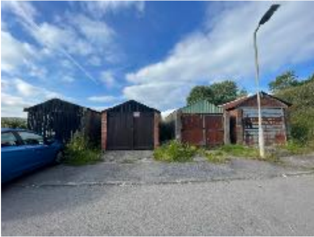
Photo 13. Garages within northeast corner of site.
