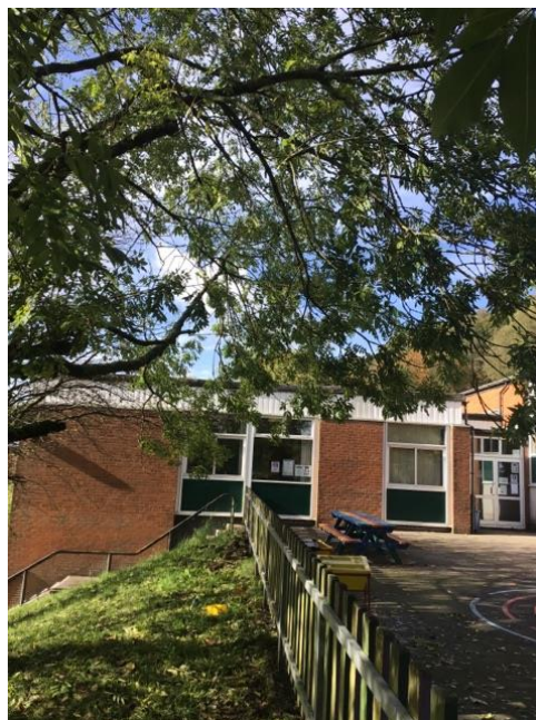
Image 6: Tree ID 2722 , Ash overhanging playground, protruding limbs to be removed to eradicate issues.
