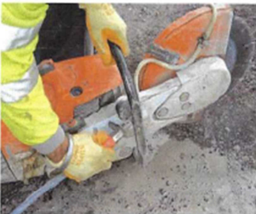
Figure 3 Water suppression on a cut-off saw
