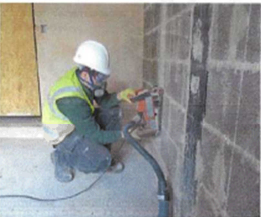
Figure 4 Wall chasing using on-tool extraction
