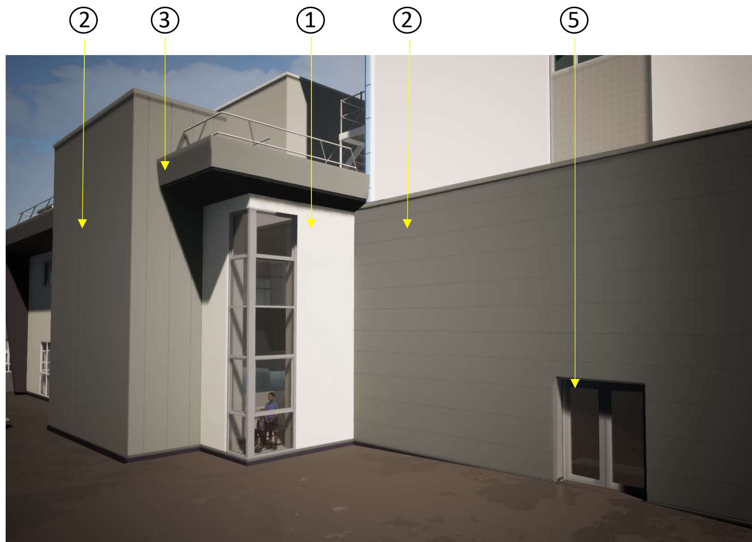
Over clad of stair core
