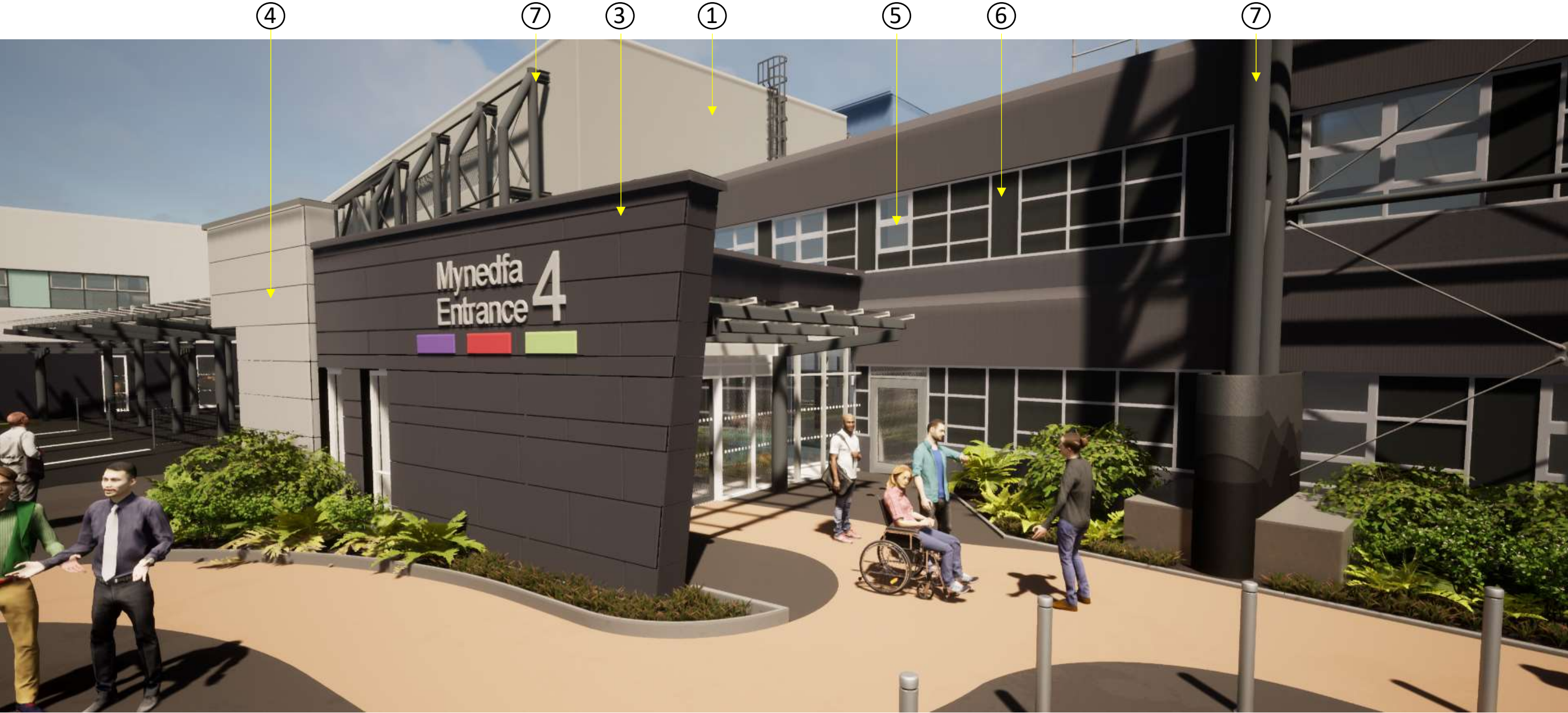
Entrance 4 – Main Entrance
