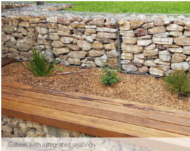
Gabion stone wall
