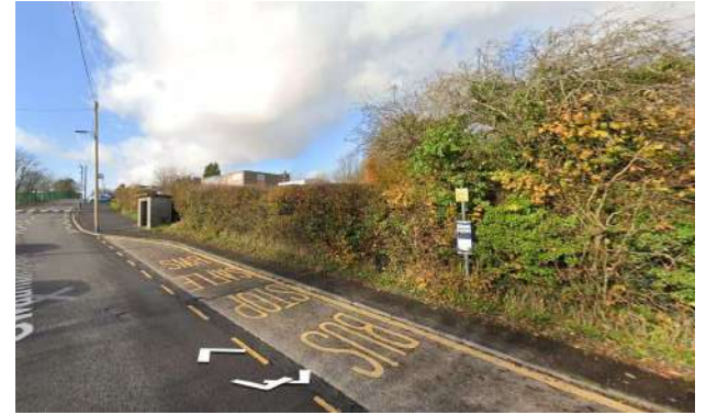
View along Gwaunfarren Rd. along layby
