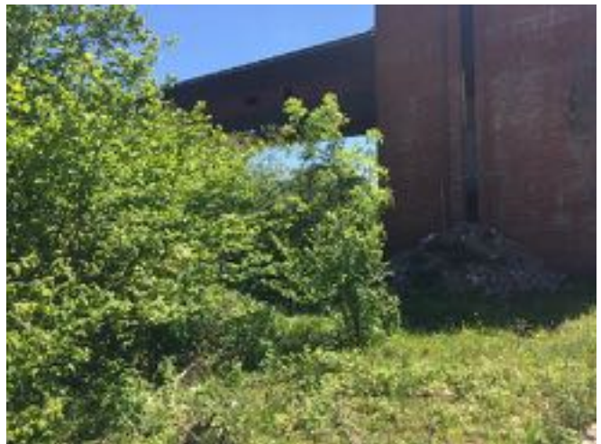
Vegetation along river at new outfall
