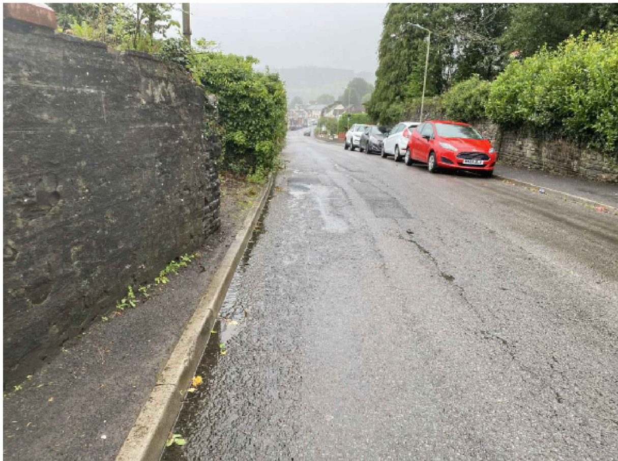
Existing Site Access View West
