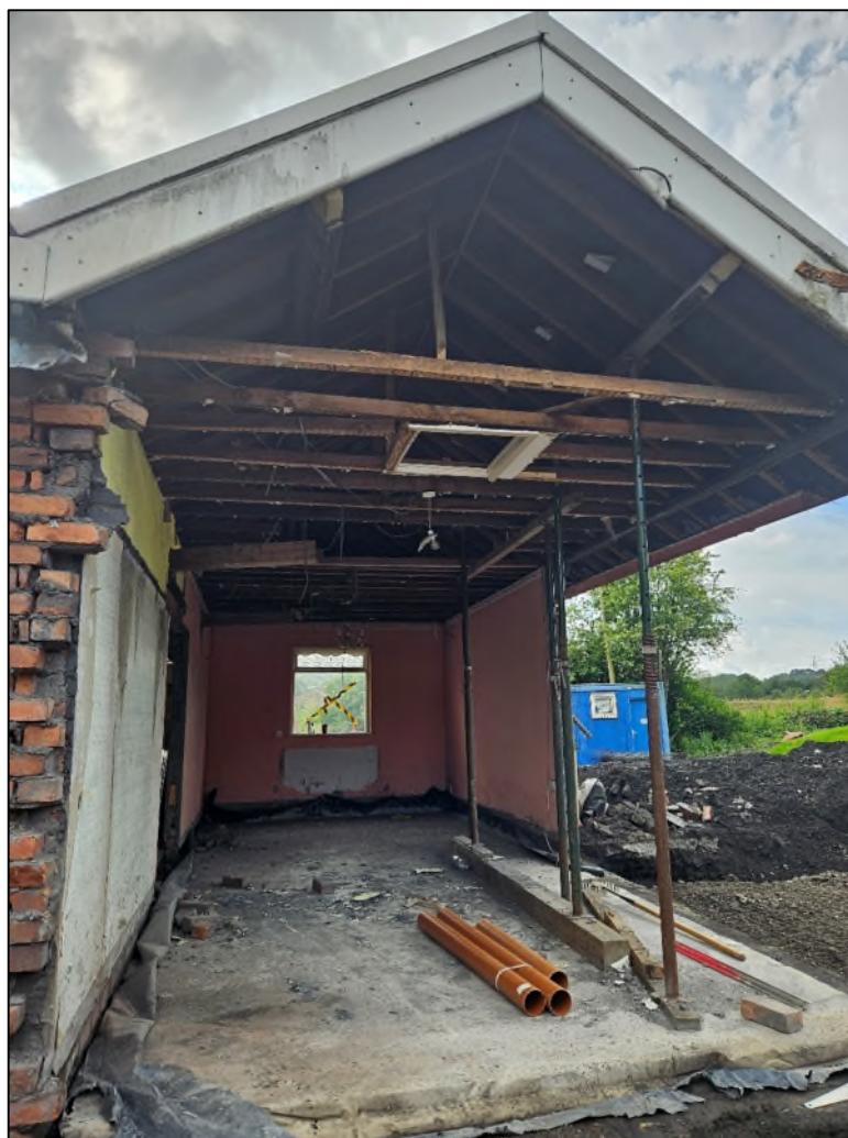
Figure 7: Inside the building
