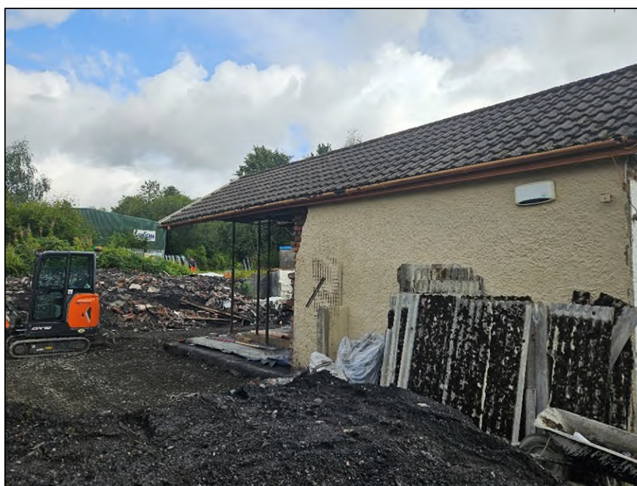
Figure 6: A view of the South side of the building with the piles of stone
