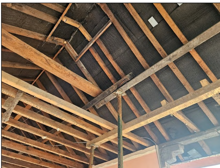
Figure 8: The roof and attic space
