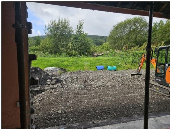
Plate 5 – The works occurring on site.
