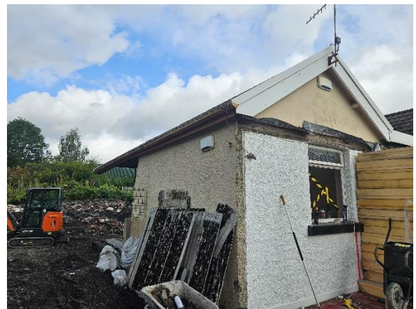
Plate 6 – The plastic soffit and fascia boards.
