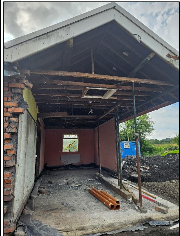
Plate 2 - The two outer walls being removed.
