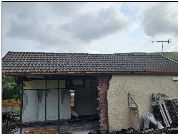
Plate 3 – The roof tiles in good condition.
