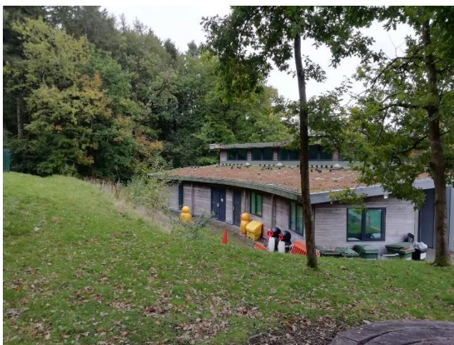
Figure 11 -Northern aspect of visitor centre, view to east
